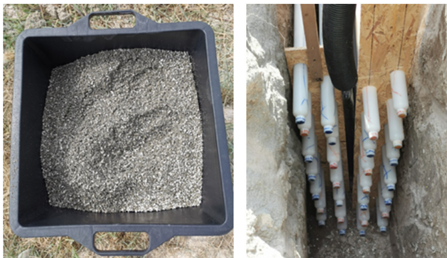
Fig. 3. Sand mixed with granules and tubes arrangement.
