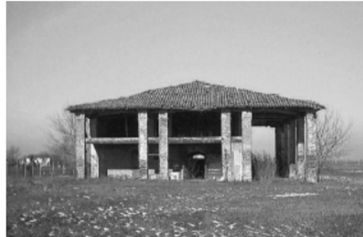
Figure 1. An example of historical rural building in the Pianura Padana territory
