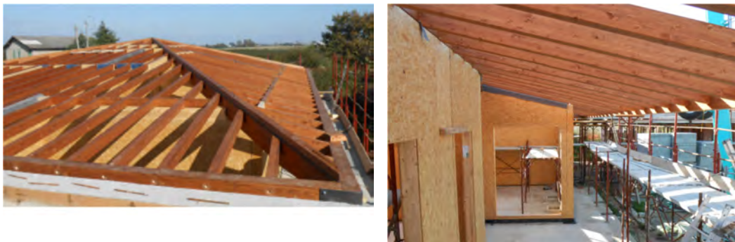
Figure 12. 8 House. The roof structure.
