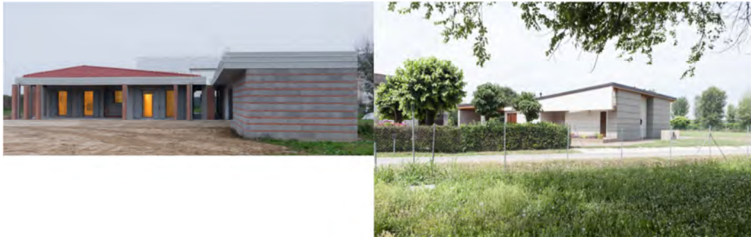
Figure 4. Case studies of modern rural buildings. 8 HOUSE, Flower House (KM429 Architects)
