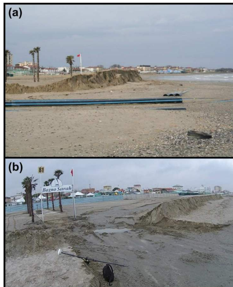
Figure 3. The state of the artificial dune at the study site of Porto Garibaldi (Comacchio, Italy) after the Saint Agatha event of 5–6 February 2015 (Photo: Enrico Duo and Edoardo Grottoli): (a) lateral view; and (b) front-lateral perspective.
