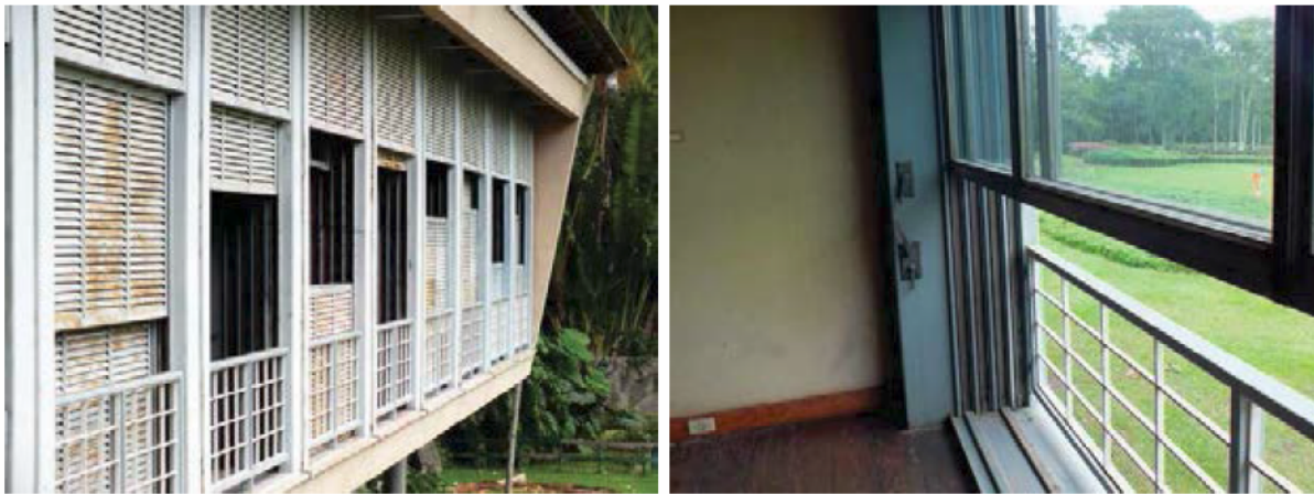
Figure 7.6: Casa Olivo Gomes by Rino Levi: the innovative window sliding system are not so easy to be restored.
