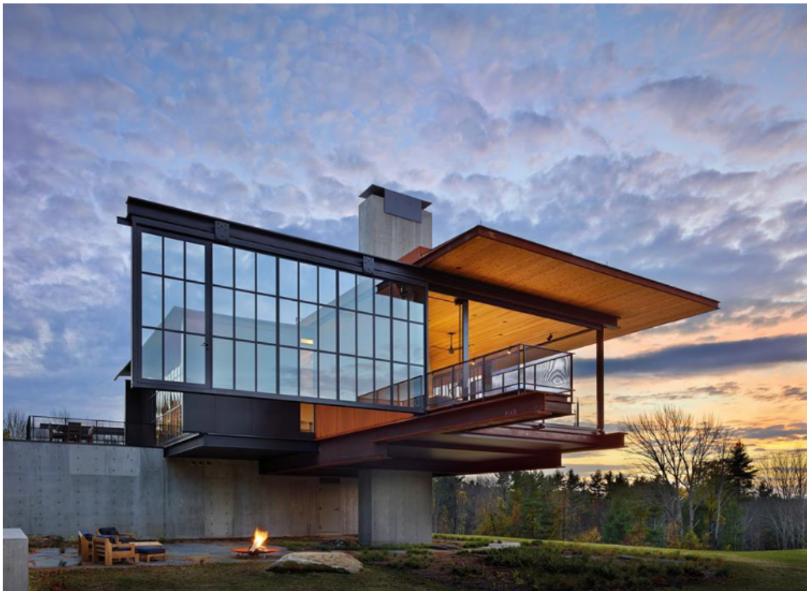
Fig. 01 – Berkshire Residence, Olson Kundig (2014), Berkshire, Massachusetts (USA). Private residence designed as low-tech smart home, symbolic of the smart definition here provided. In this project indeed, facades can transform without recurring to advanced technologies but just employing a complex system of cranks and levers.
