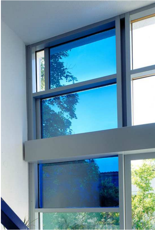
Fig. 42 – Gasochromic glass, installed at Fraunhofer ISE
