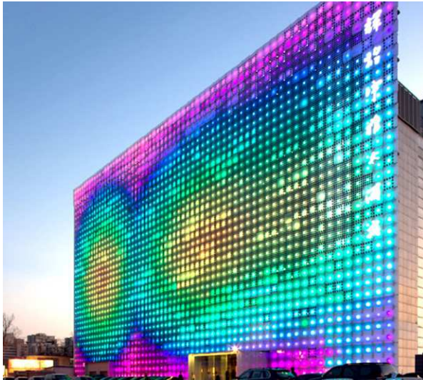
Fig. 11 – Examples for media façades with adaptive functionality: Green Pix Zero Energy Media Wall uses photovoltaics for the needed energy, Beijing, China, by Giostra & Partners
