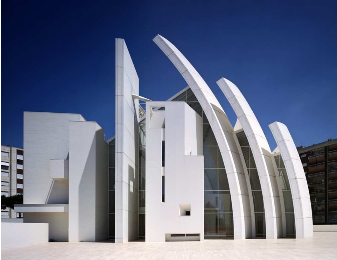
Fig. 05 – Jubilee Church, R. Meier & Partners, Rome (1998-2003). The photocatalytic concrete cladding, with Carrara's marble aggregates and titanium dioxide, allows the activation - in presence of natural lighting – of an oxidative process able to decompose organic compound, further removed thanks to the washing away of rainwater.
