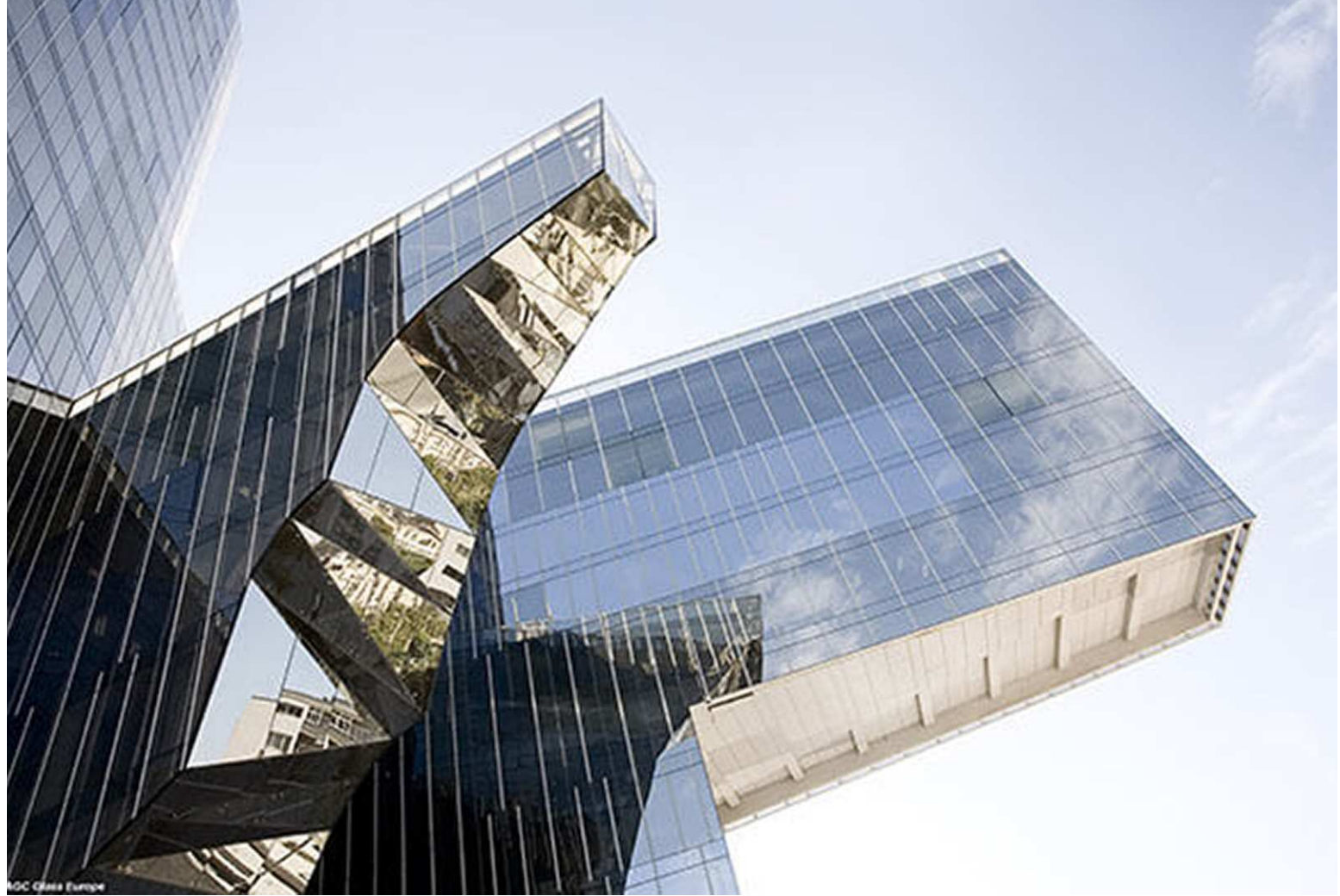
Fig. 04 – Office building with reflective glasses for solar control.
