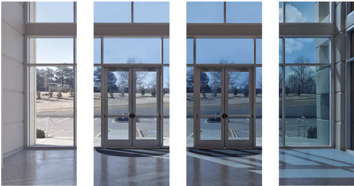
Fig. 31 – From left to right, electrochromic windows under different operation mode.
