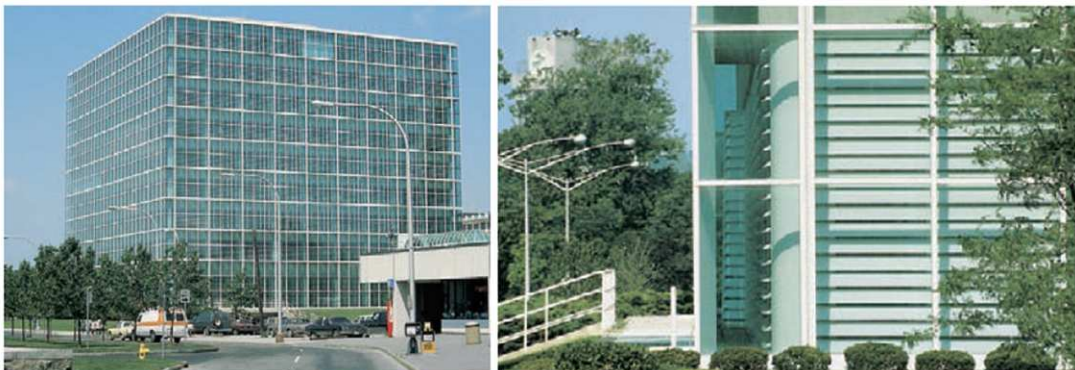
Fig. 06 – Cannon Design, The Occidental Chemical Building (1981), already known as the Hooker Building at Niagara Falls, New York; it is one of the first buildings which incorporate intelligent responses in its skin. The protecting louvres indeed, tilt automatically to keep the sun's direct beams from striking the internal glass wall thanks to the action of a solar cell on one louvre on each bank.
