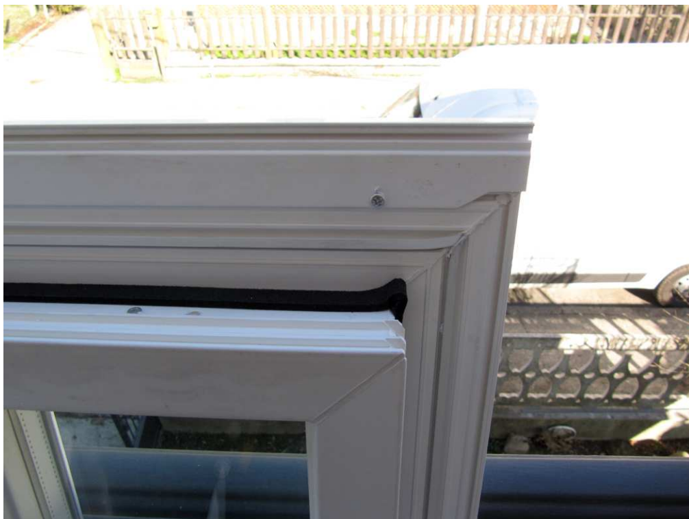
Fig. 07 – Application of auto-expanding tape on a window frame
