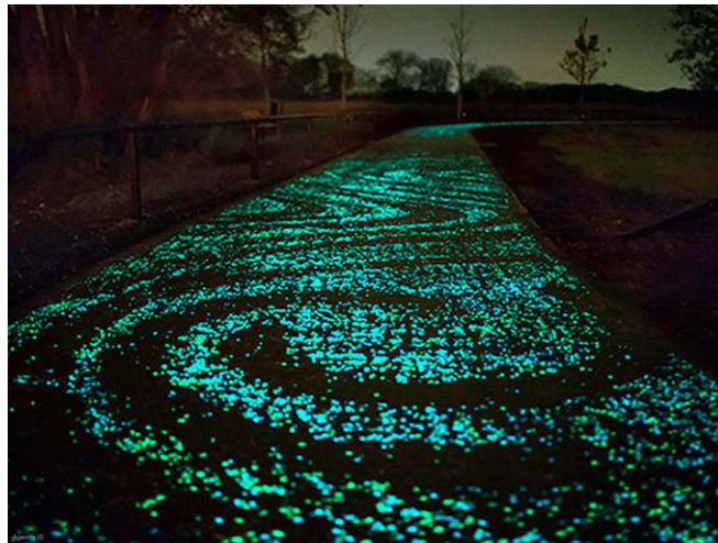
Fig. 06 – Fluorescent concrete.
