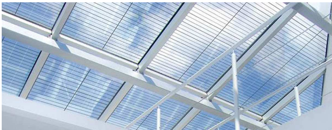
Fig. 23 – Semi-transparent PV modules
