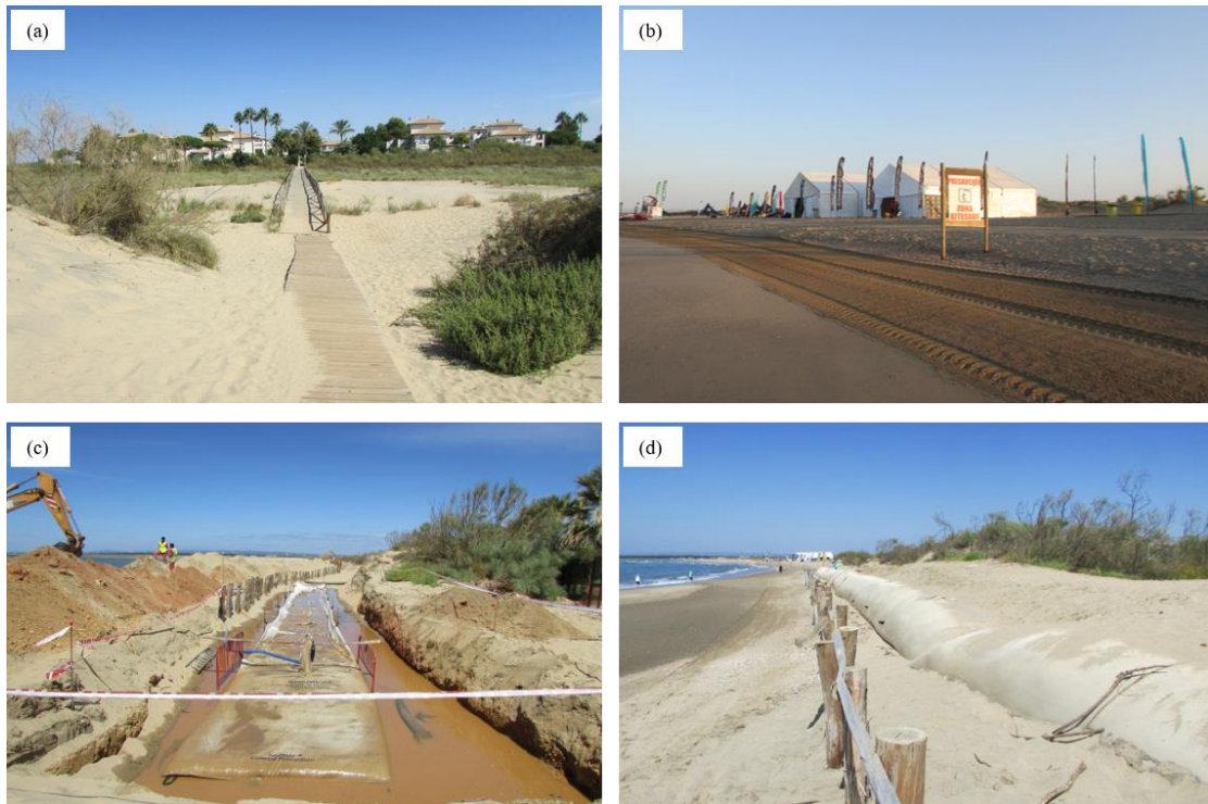
Figure 6.22. (a) Access path to holiday buildings, (b) information panel situated on T6, (c and d) sand collectors in Guadiana estuary.
