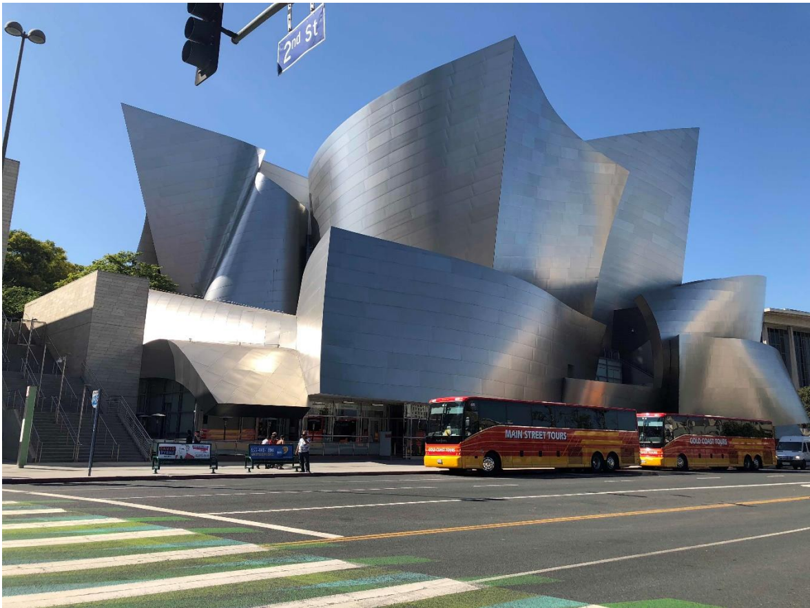
Figure 38 Gehry's Walt Disney Concert Hall (2003) demonstrates how buildings have become increasingly complex and non-standard. Photo: Khalid Salih
