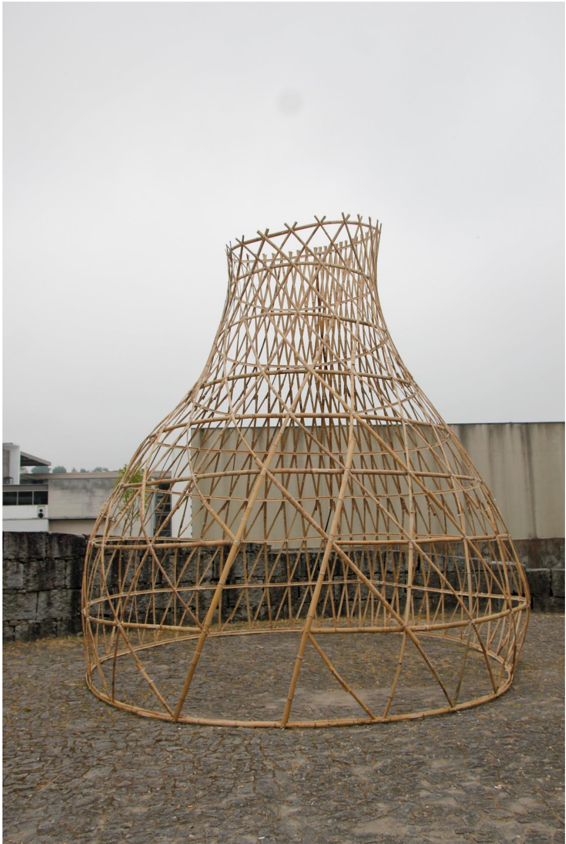
Figure 94 Finished bamboo structure. Photo: Jona Rapi (2018)
