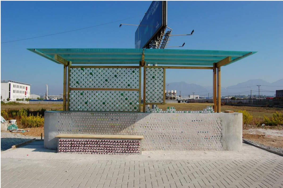
Figure 18 Plastic Bottle Bus station built near Polis University during the first edition of Tirana Architecture Weeks. (2012)
