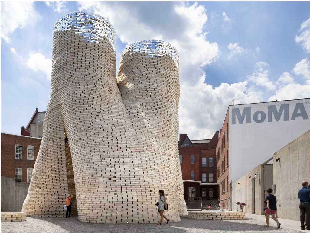
Figure 30 A collaboration of New York-based architects Hy-Fi is a cluster of brick towers grown from mushroom at MoMA's PS1 venue, source: The Living (2014)
