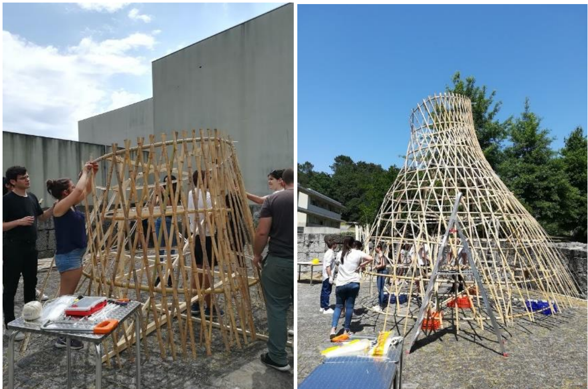
Figure 91 (a) assembly of the first part, placing bamboo strips (c) Assembly almost finished with all three parts photo: author (2018)
