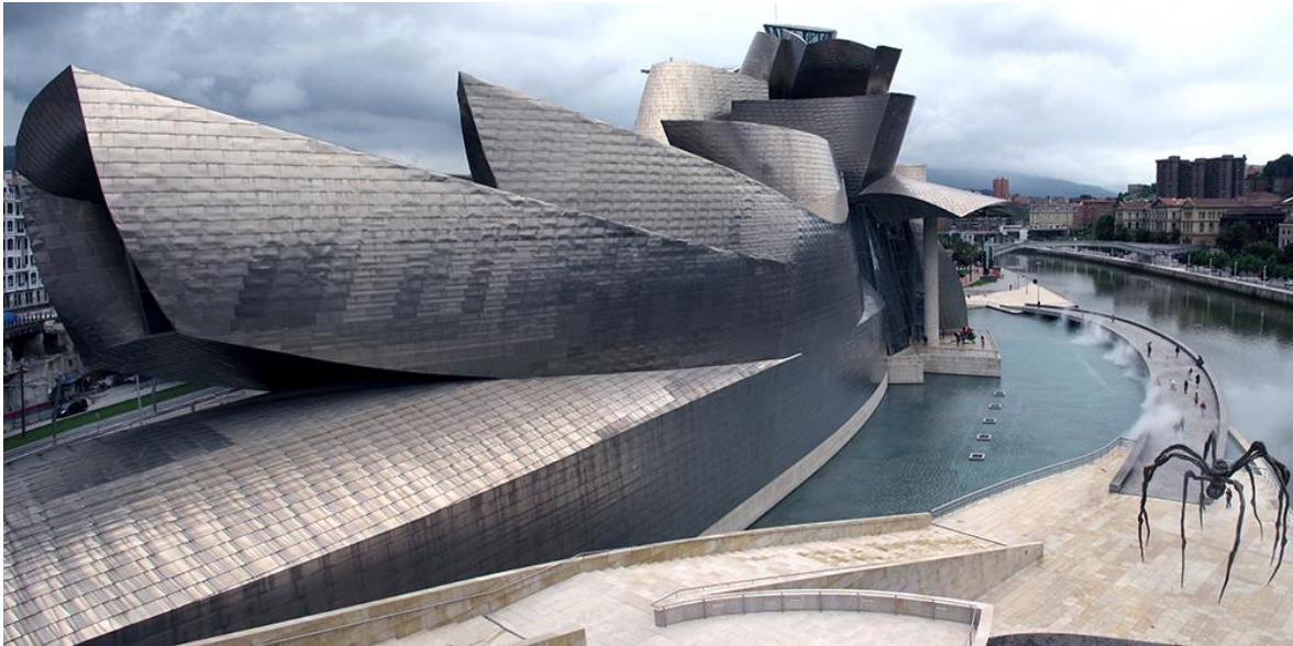
Figure 47 Guggenheim Museum in Bilbao by Frank O Gehry (1997) was made possible through directly fabricating design information. Photo: Emilio I. Panizo
