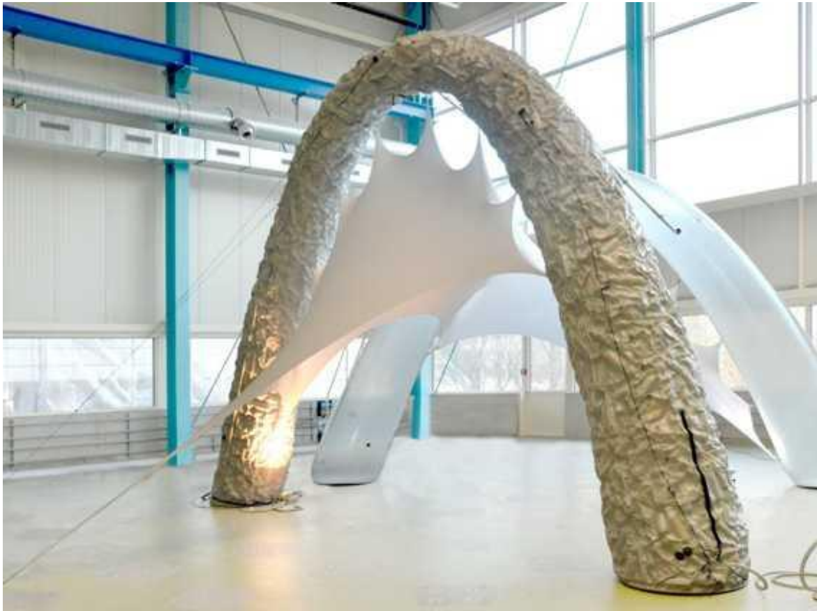
Figure 22 Airless, a pavilion built out of compressed PET bottles enclosed in a membrane, source: ETH Zurich (2014)
