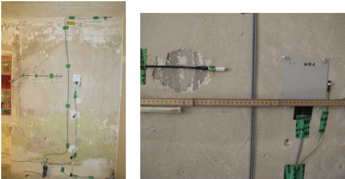
FIGURE 29 - SENSOR SET UP ON THE TRANSIENT LAYER, RIGHT OF THE WINDOW REVEALS: CAPACITIVE SENSOR, HEAT FLOW METER AND TEMPERATURE SENSOR (IMAGE COURTESY OF FRAUNHOFER)
