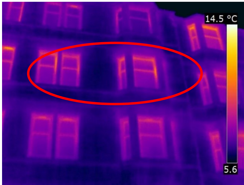
FIGURE 24 - INFRARED IMAGES OF THE BUILDING TAKEN FROM OUTSIDE
