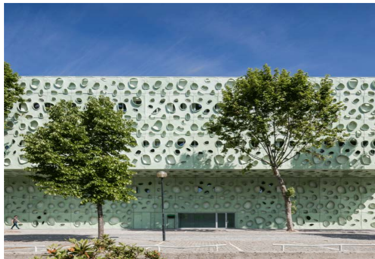
Figure 2.5.19. The exterior perforated concrete wall of University science institute at Portugal
