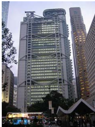
Figure 2.2.5. The HSBC Hong Kong headquarters
