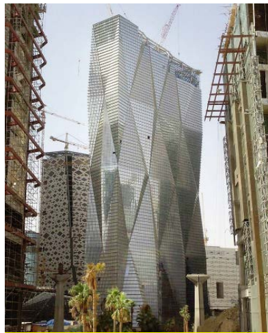
Figure 2.2.4. Gallery of Muqarnas Tower by SOM, Saudi Arabia
