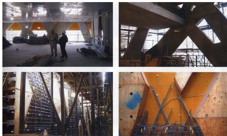
Figure 2.5.10. Criss-crossed concrete braces skin of TOD's Omotesando Building, Tokyo
