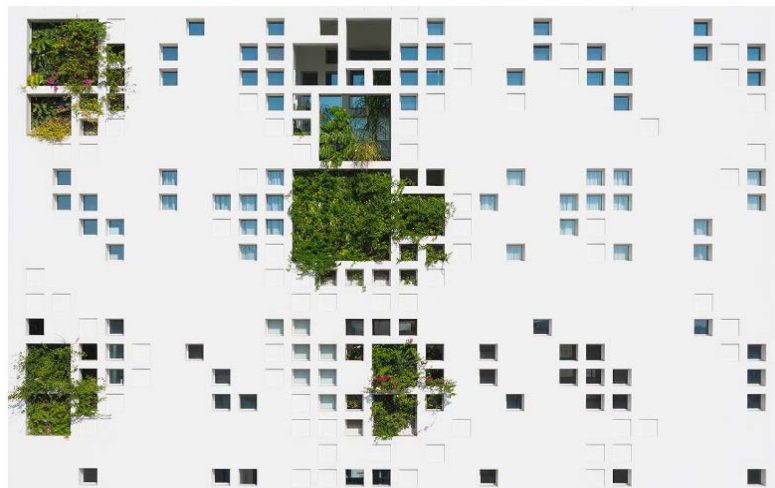
Figure 2.5.16. The exterior perforated concrete wall of Jean Nouvel’s Cyprus Tower
