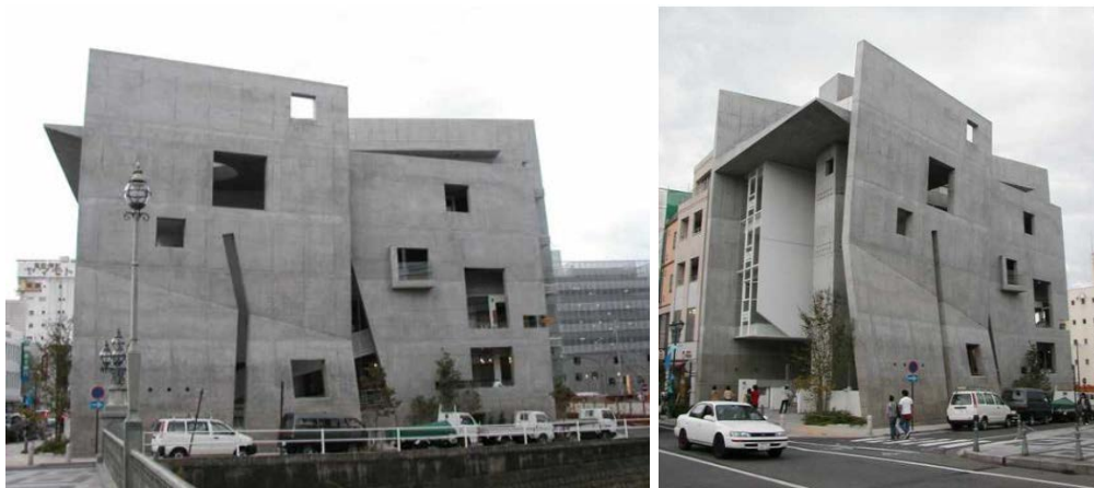
Figure 3.4.1. Building in Nagano, Japan, with vertical extension - unusual Structural Walls (source: Llundji, 2012)
