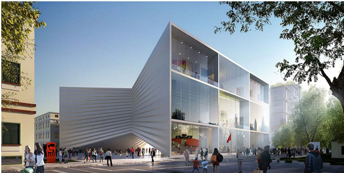
Figure 27. [Above] the Ensemble of the National theater. Tirana. 2018. Photo credit Tsai Mali. [Below]The bow tie shaped project form Bjarke Ingels. Photo Credit: Bjarke Ingels group
