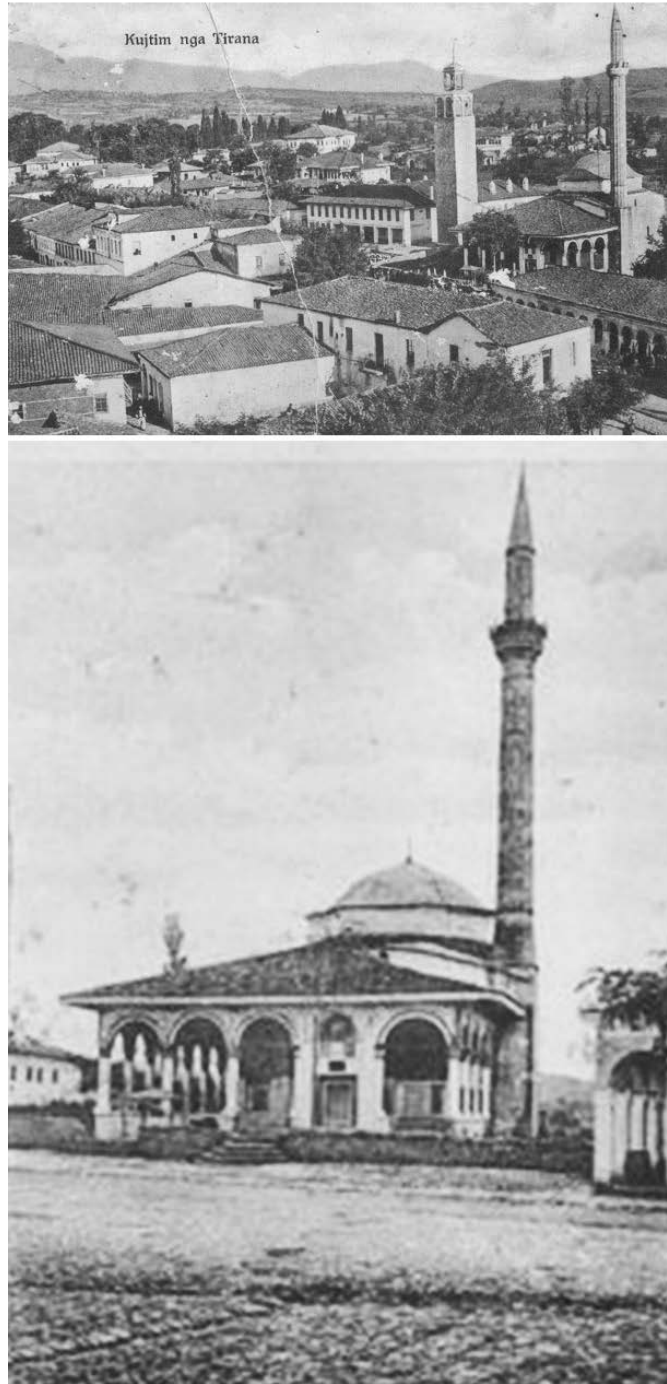
Figure 44. “The Ethem Bey Mosque”. (Above) The Building is shown with its surrounding context; the hills in the background are toward the road to Elbasan, traveled in the first part of the itinerary. The photo was probably done from the minaret of the Terzi (karapici) mosque. (Below) The Front of “The Ethem Bey Mosque” with all its elements visible. Tirana: Aprox. 20s. Old postcards.
