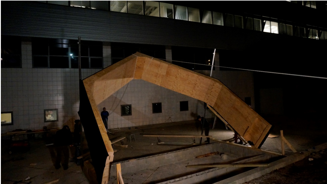
Figure 20 - Jacking first section onto the foundation
