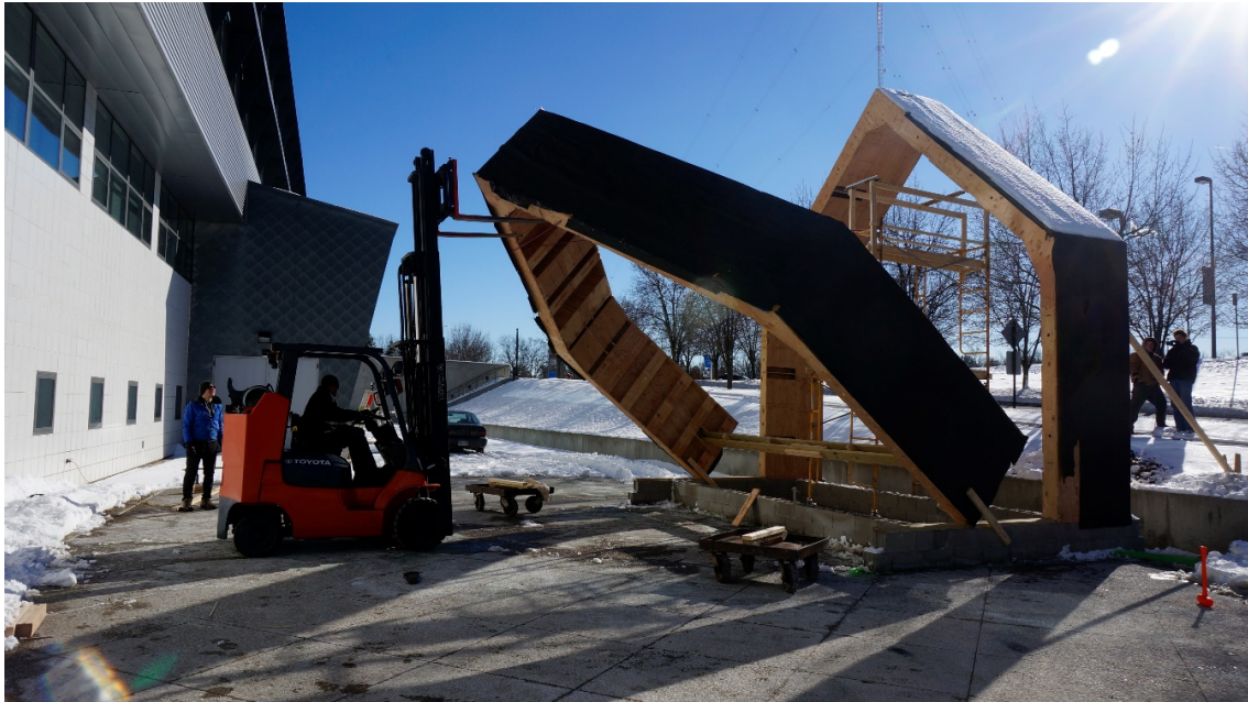
Figure 21 - Hi Low lift used for safety during jacking
