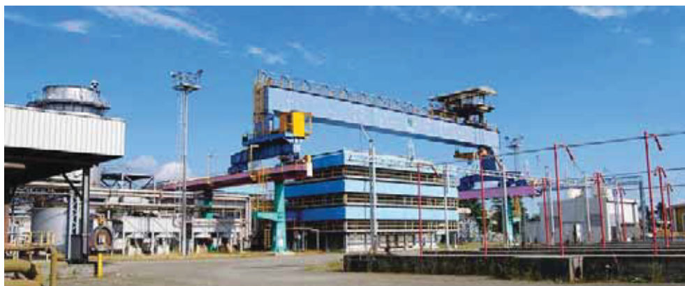
Fig. 266 Alessandria power plant (source: Enel)
