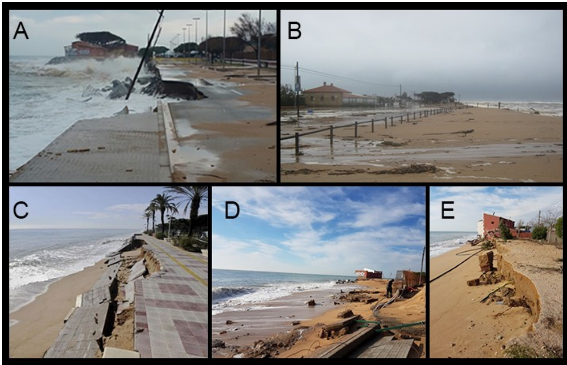
Figure 6.2 Impacts on the Tordera Delta. Destruction of a road at Malgrat (A); overwash at campsites north of the river mouth (B); destruction of the promenade north of the river mouth (C); beach erosion, and damage to utilities and buildings at Malgrat (D and E).
