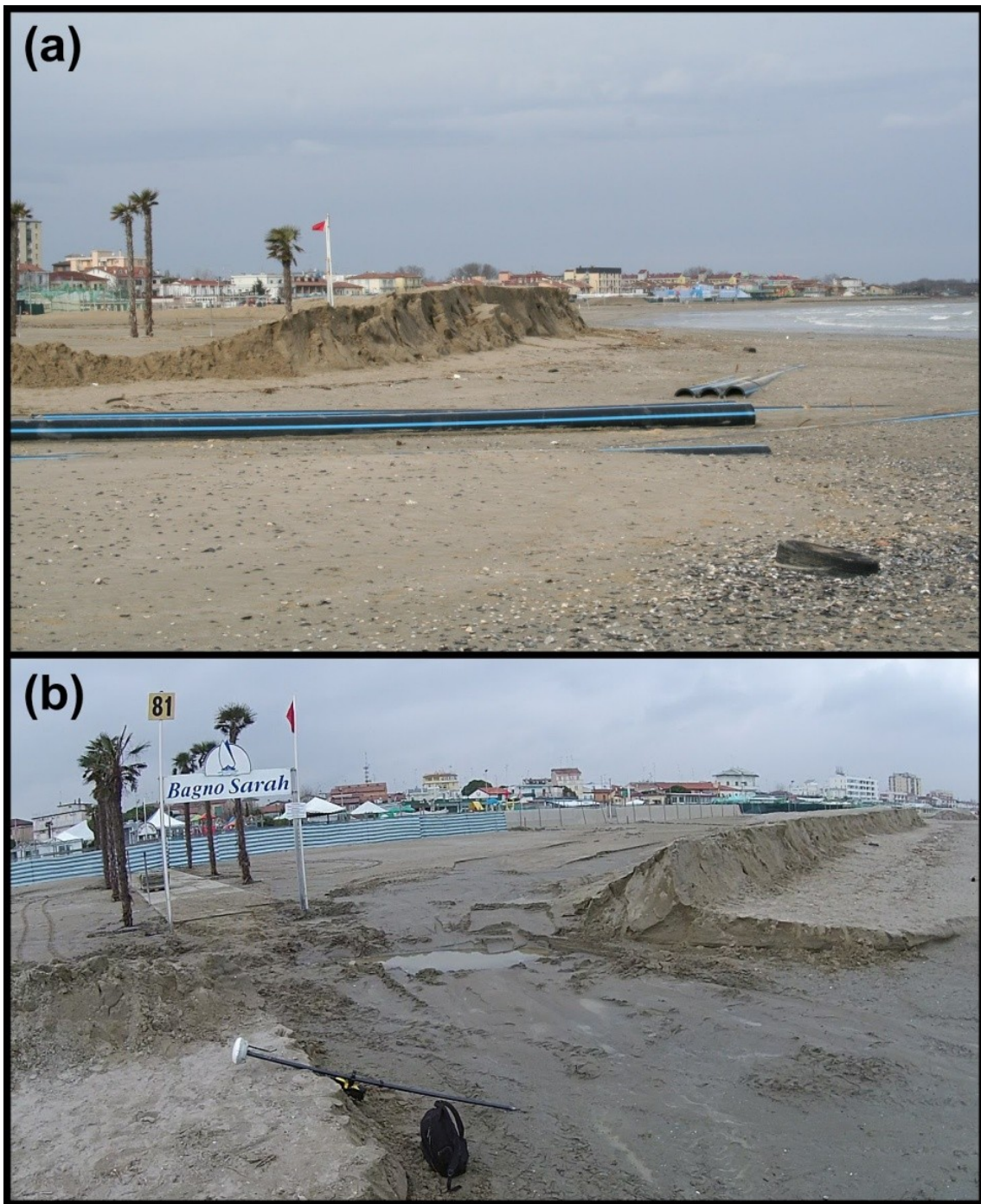
Figure 3.2 The impacts of the Saint Agatha event of 5-6 February 2015 on the artificial dune at the study site of Porto Garibaldi (Comacchio, Italy).
