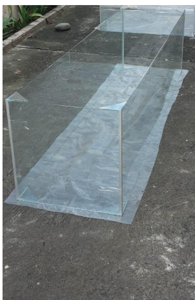
Figure 16 Pilot station construction VSSF CW
