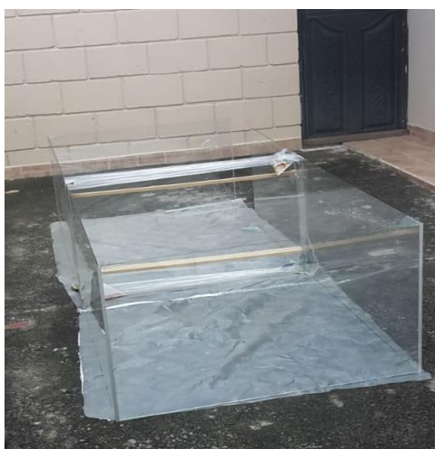
Figure 15 Pilot station construction HSSF CW
