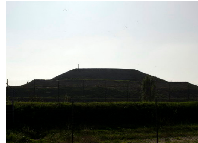
Fig. 122. Ravenna (Italy). Landfill in wooded area. In a urban landfill waste is stored and isolated from the ground through soil sealing works. At these sites the soil is impermeable even if the landfill is coated with earth and plant material in order not to disperse polluting materials in the soil. Anyway they are considered effective land take.
