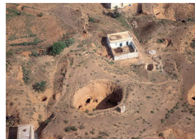
Fig. 105. Matmata (Tunisia). Dwelling consisting of a pit courtyard dug out of clayey soil. The rooms overlooking the courtyard have underground connections with others of the same kind. A pit-courtyard acts as an impluvium and provides an open-air sunny space, surrounded by walls. Some of these courtyards are used for collecting waste and produce humus, and form gardens carved out of the rock. This technique solves the problem of soil infertility and the need to protect plants.
