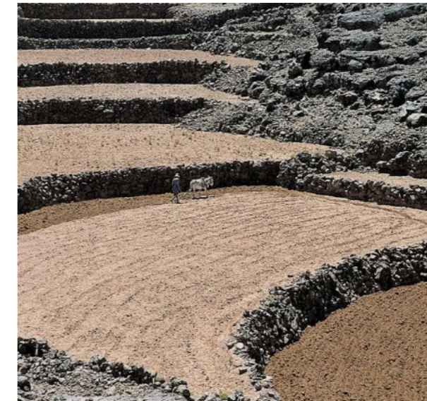
Fig. 81-82. Right: Yemen. Above, at the bottom of the marbid the stone walls which organize the terraced slope and collect humidity. source: The water Atlas, Laureano.
