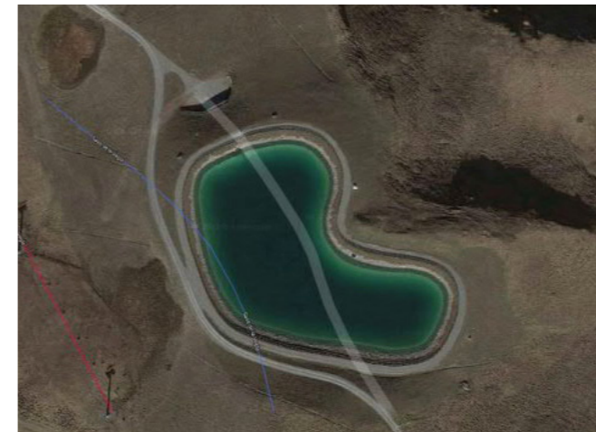
Fig. 104. Val di Fassa (Italy) Controlled snow-making system and reservoir in case of snow lacking. The need to have artificial snow basins requires the excavation of large waterproofed areas with material repositioning on site. The levelling of slopes allows water to be conveyed into the excavated basin.
