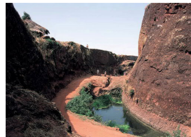
Fig. 123. Lalibela (Ethiopia). Deep ditches surround the underground monumental complexes of Lalibela. Their water drainage and harvesting function is proved by the reservoirs for conserving the precious liquid in the dry seasons. Urbanization progresses according to this hydro-agricultural pattern by saturating the sloping terraces with constructions or turning the fields in the valleys irrigated by stream-roads into squares surrounded by buildings.
