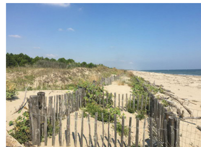
Fig. 108. Ravenna (Italy). Dune setting re-naturalization in Lido di Classe in a protected area. Topographical conditions are created with the help of wooden piles so that the sand spontaneously settles along the damaged dune belt. The process is slow but follows the course of nature in the sand deposit that is shaped by wind and vegetation.
