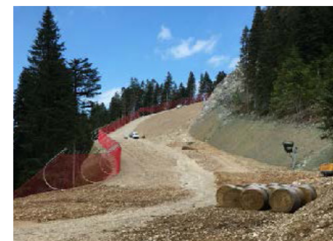
Fig. 111. Andalo (Italy). The development of ski facilities has completely re-designed the morphology of the mountain sides to make these areas accessible to tourists. This involved in addition to massive deforestation, the reshaping of slopes using reinforced soil walls and slope reinforcement.
