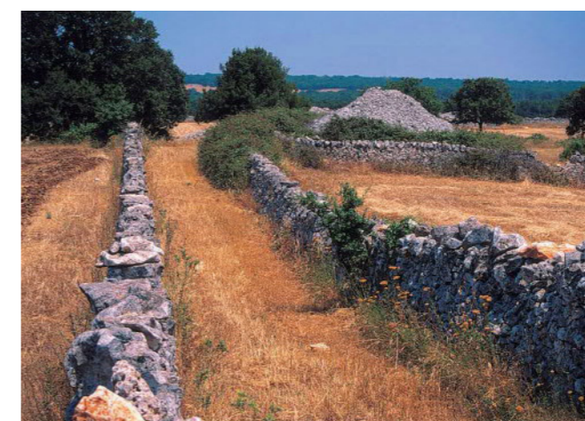
Fig. 126. Apulia (Italy). The dry stone walls and the "specchie" of the Apulian countryside constitute a titanic landscape-organizing work, useful for catching moisture and maintaining the hydromorphic capacity of soil.
