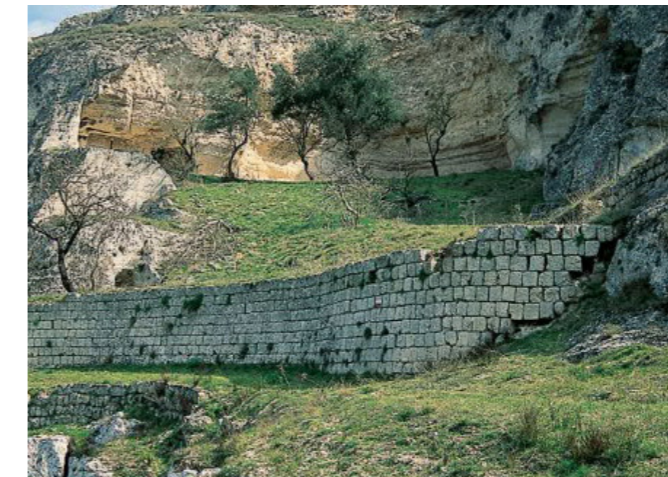
Fig. 110. Matera (Italy). Massive dry stone walls protect from the effects of the rainfalls and create the space for cultivations organised on artificial terraces along the slopes of the Palomba of Matera. Matera boasts the Sassi, a primeval ancient site where the Neolithic ditches and the agro-pastoral terracing system attest to the ways of inhabiting the caves and managing the soils.
