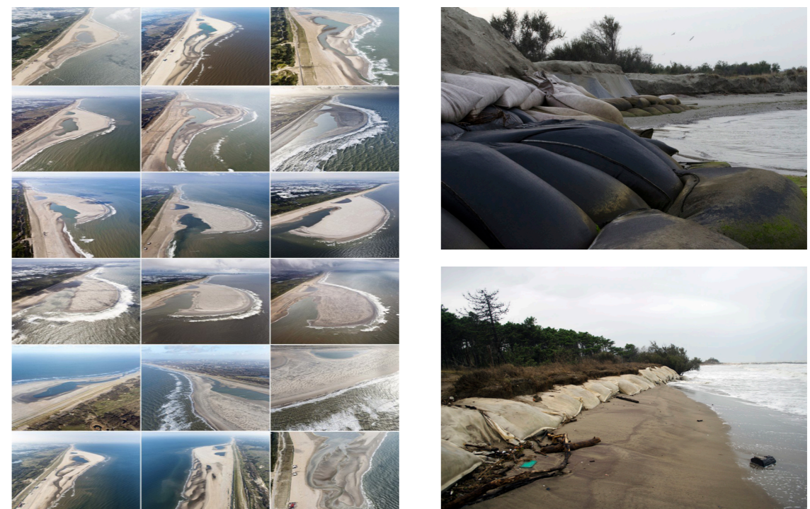
Fig. 52-53. Dynamic and rigid coastline. On left a sand engine in the Netherland. source: “Understanding sediment bypassing processes through analysis of high-frequency observations of Ameland Inlet, the Netherlands”, Elias, 2019. On the right coast line defense in Lido di Spina (Italy), source: author
