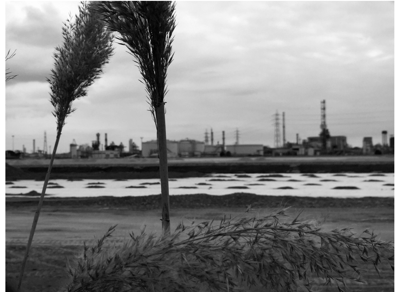
Fig. 29. Construction site of special waste landfill in Ravenna, 2021. source: author
