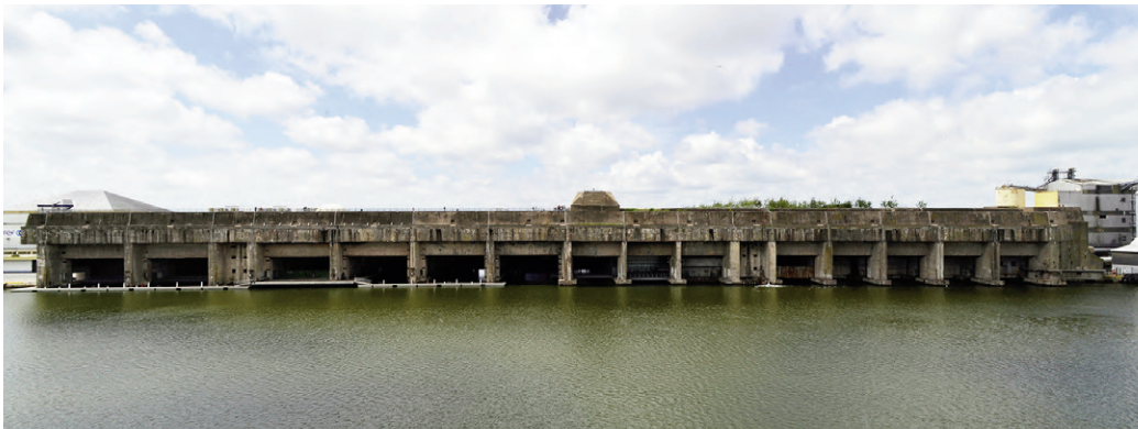
Fig. 1 | The submarine base of Saint-Nazaire, Alvéoles 12-14 (source: commons.wikimedia.org, 2012).
