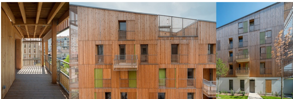
Figure 2.12 Case 2- Paris housing blocks by Tectône Architectes
