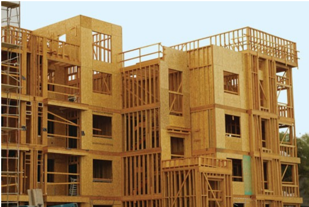
Figure 2.9 Case 1- Exterior view during construction phase
