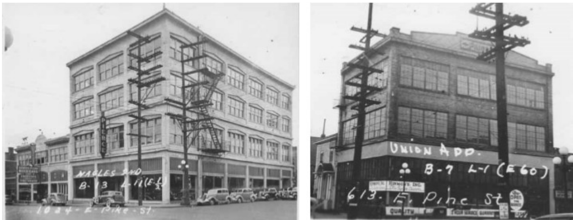
Figure 2.3 Left - Four storey timber building in Seattle, constructed in 1913, still in use; right - three storey timber building in Seattle, constructed in 1917, still in use
