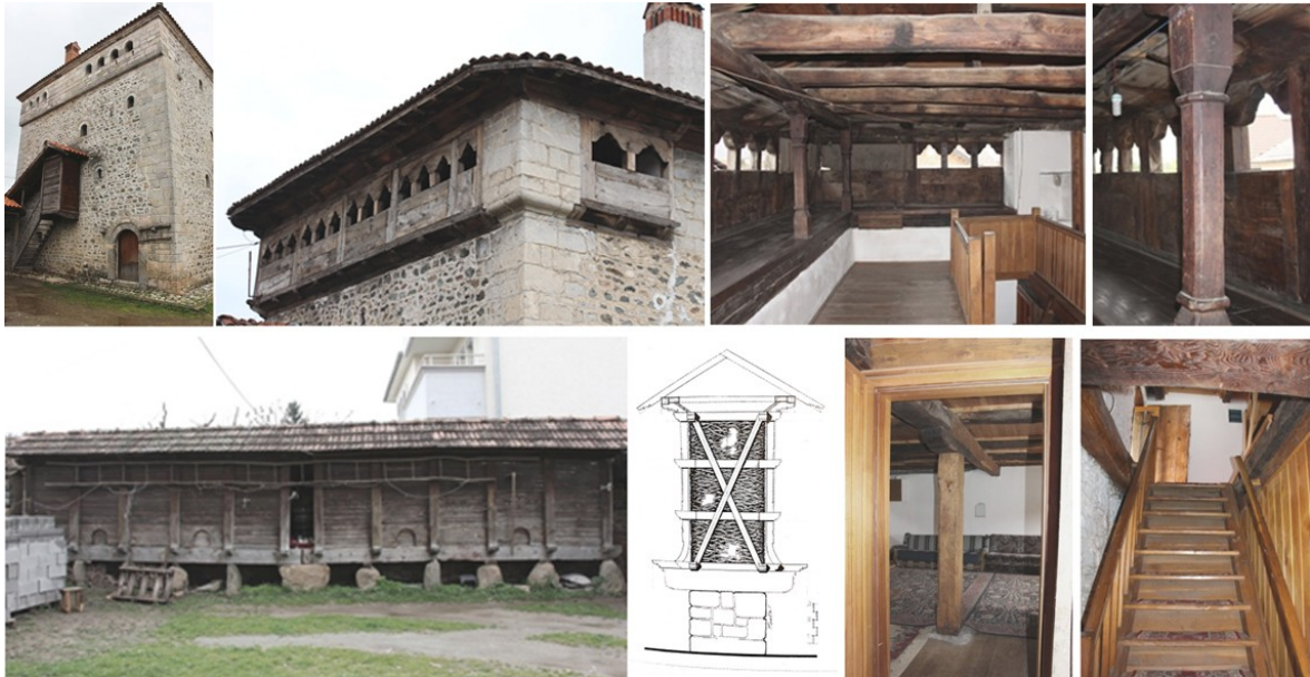
Figure 3.30 Wooden elements of Kulla and Corn sheds in the complex; drawing in lower row (Doli, 2001)
