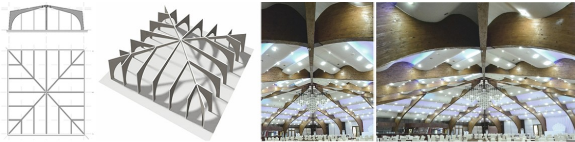
Figure 3.31 Large span glue laminated timber structure, Pejë
