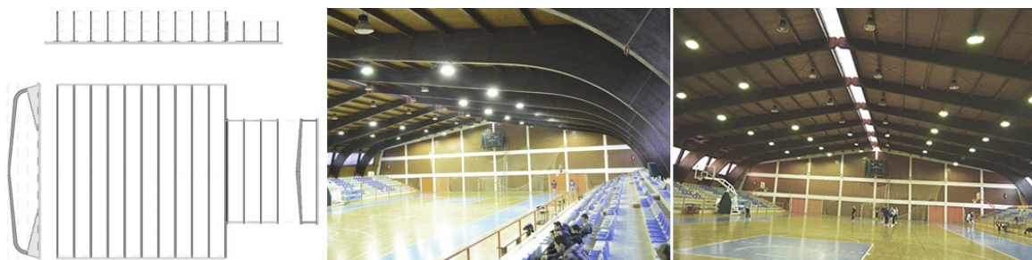
Figure 3.32 Large span glulam timber structure, Vushtrri
