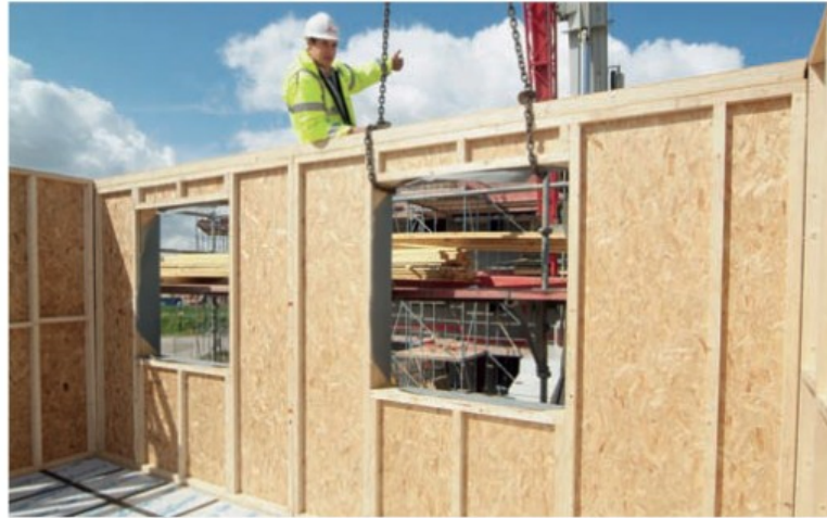
Figure 2.29 Case 7 - Panel wall assembly.
