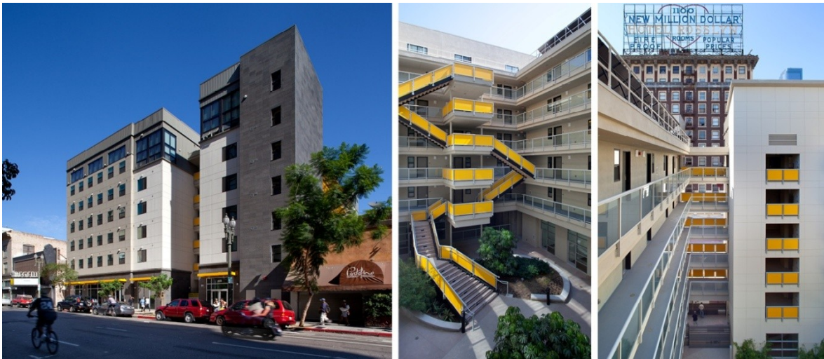
Figure 2.8 Case 1-Exterior view; Genesis Apartments in Los Angeles, CA
