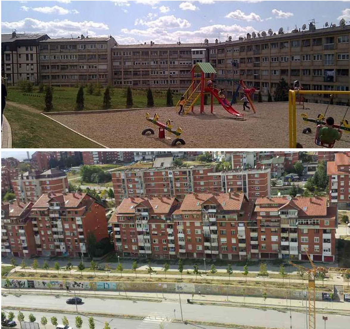
Figure 3.10 Mid-rise residential blocks in Prishtina
