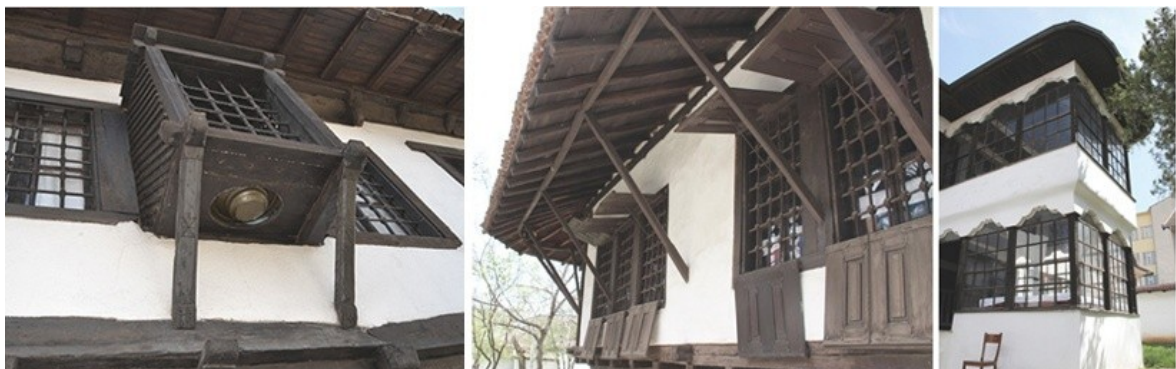
Figure 3.24 Wooden exterior structures; Source: Author
