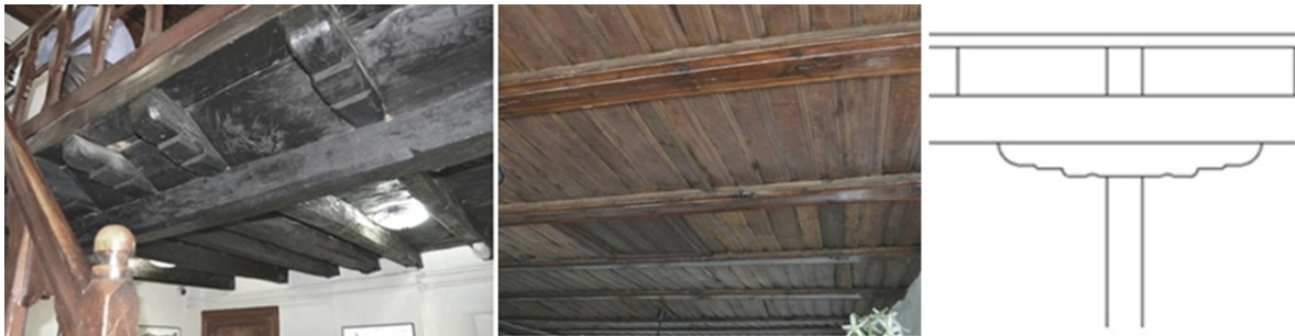
Figure 3.21 Timber beams, Source: Author
