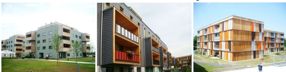
Mid-rise timber-based residential buildings. Photo: Arta Januzi-Cana
