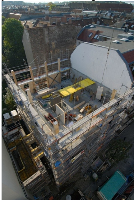
Figure 2.16 Case 3 - Exterior view during construction
