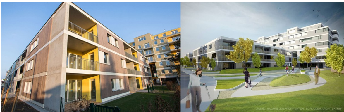
Figure 2.20 Case 5 - Exterior view
