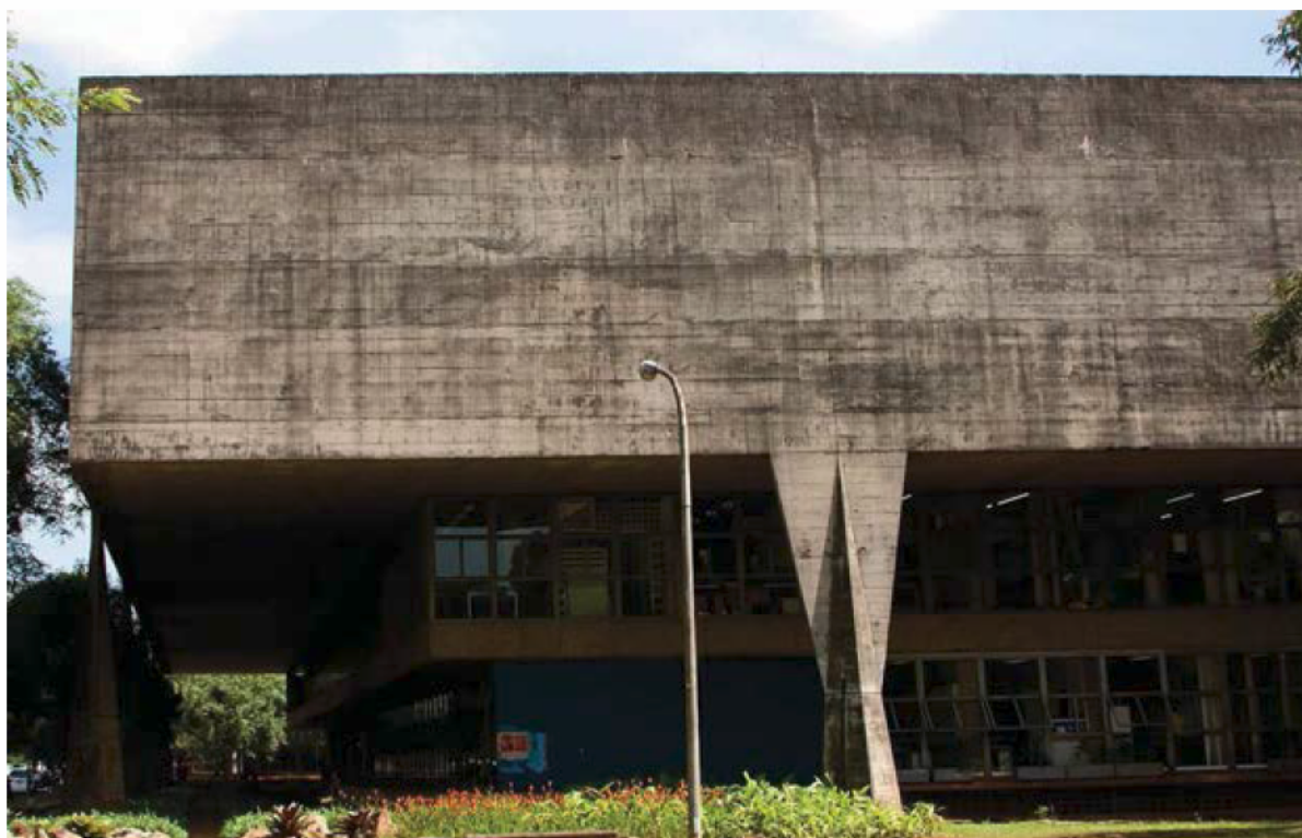
Figure 8.12: FAU USP building, one of the façades before restoration in 2014.
