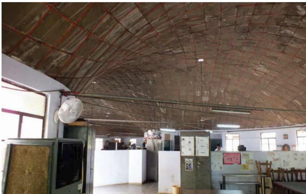
Figure 9.6: Internal view of vaulted ceiling in April 2016.
