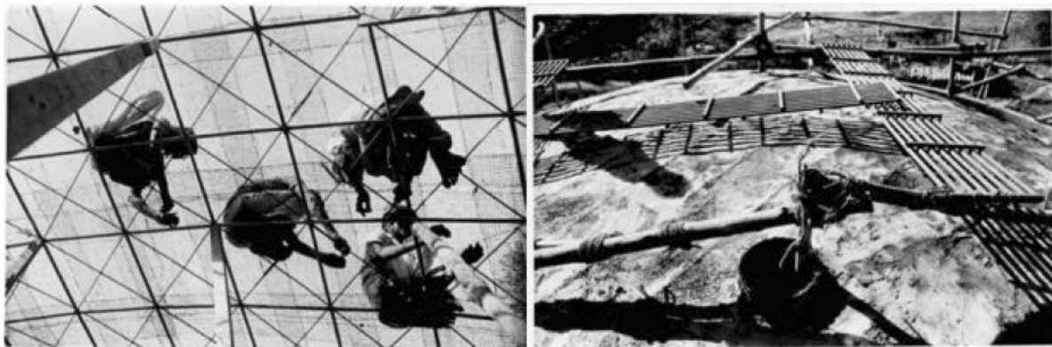
Figure 9.3: Two construction phases of the dome.
