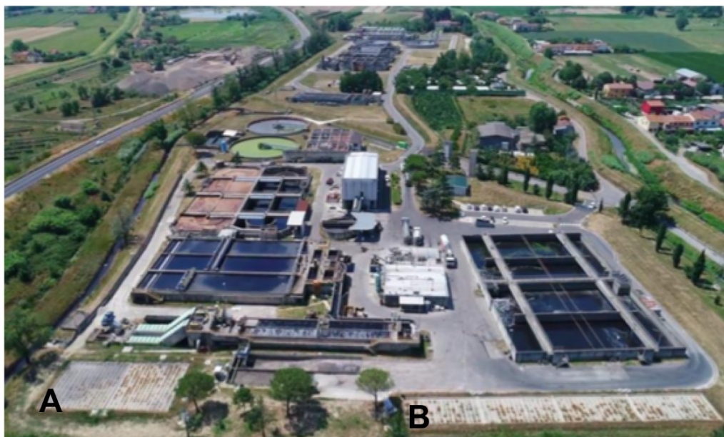
Figure 16. Calice WWTP in Prato. A / B indicate the vertical flow CW flow CW.
