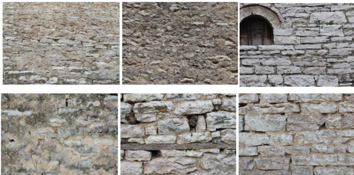
Fig. 149 Buildings masonry material and texture samples made of limestone (source: author's)
