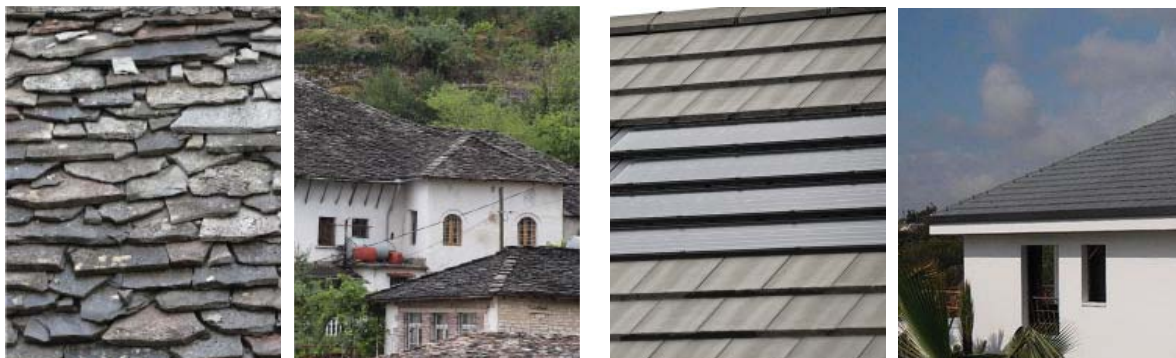
Fig. 148, Visual integration of roof color and texture in new design. Existing and possible proposed design of the roof in the residual area (or buffer zone) (source: author's)
