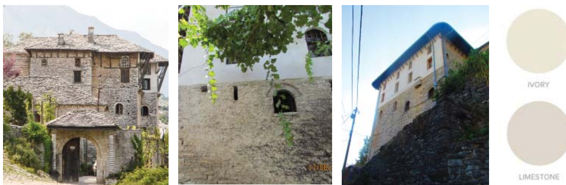
Fig. 150, Visual integration of masonry surfaces. Existing masonry facades and possible proposed design facade colors or materials for in the residual area (or buffer zone) (source: author's)
