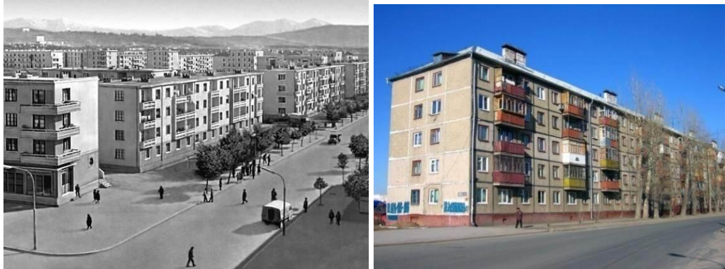
Photo 1 Similarity in different region Street “21 Dhjetori” , Tirane. Year's 70 second picture panelled building in Russia year 60'
