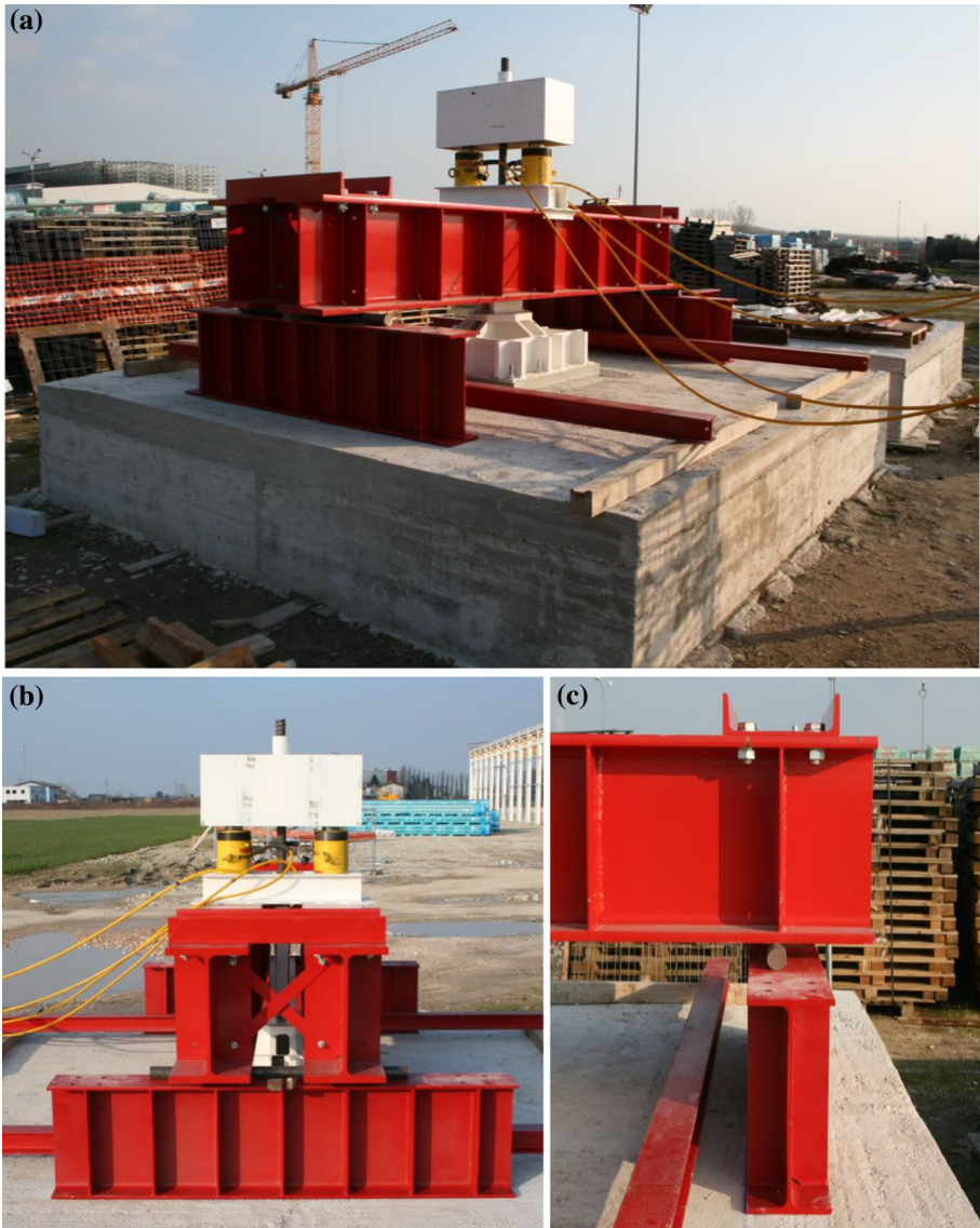
Fig. 12 Setup for tests on anchor groups: a overall view; b front view of test rig; c detail view of one of the supports of the reaction frame
