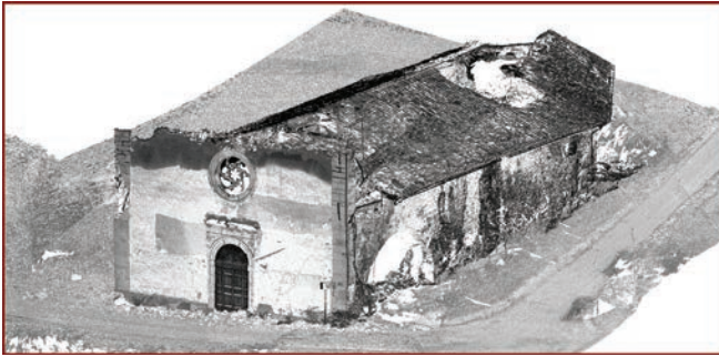
Figure 10. Laser scanner point cloud of Sant'Andrea Church.
