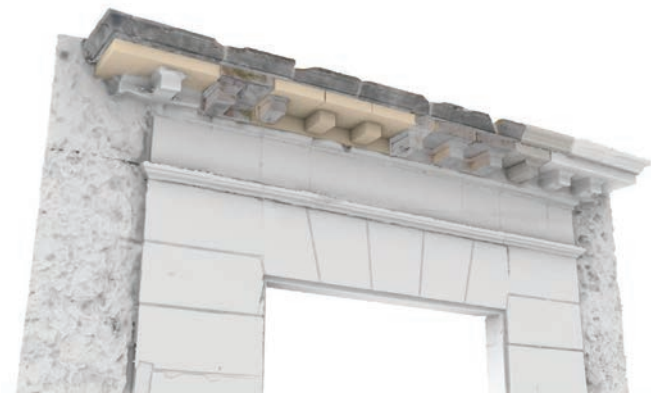
Figure 13. The virtual re-collocation of the elements recognised in the rubbles of Palazzo del Governo (AQ). The different colours identify the elements still in situ, the elements virtually re-located and elements definitely lost which are represented through simplified forms.
