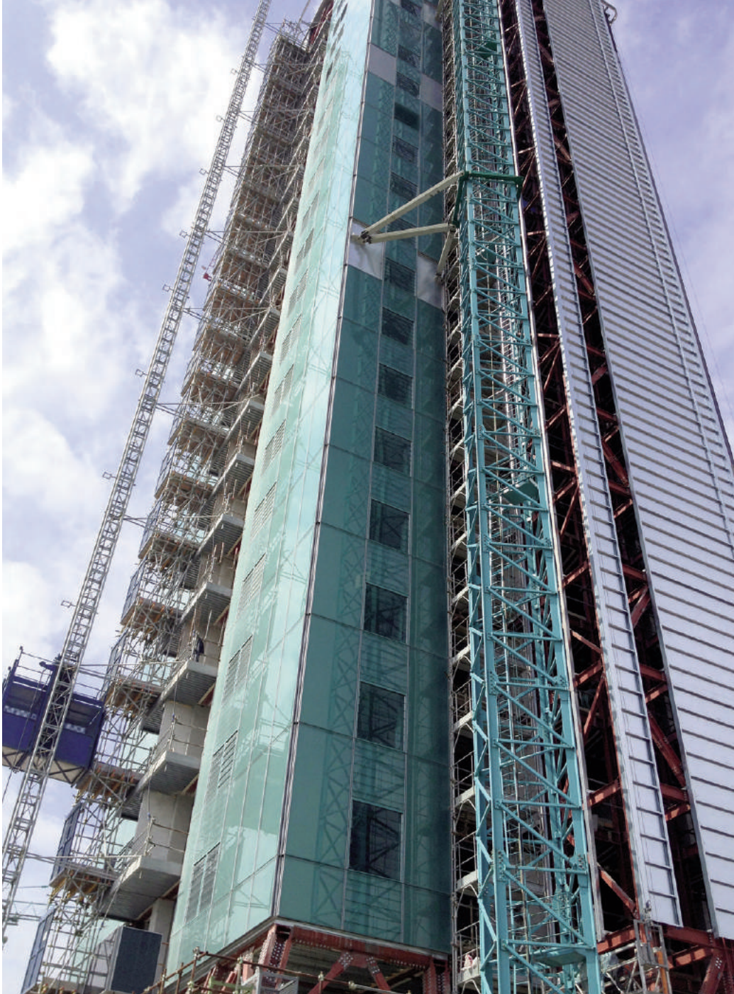
Fig. 5 | Residential Tower in Castelmaggiore (Bologna), during the construction phase of the double-skin glass facades. Building's general features: 7,000 sqm of built surface, n. 90 apartments, n. 1 commercial structure, n. 1 restaurant, n. 1 Spa, offices (credit: F. Conato and V. Frighi).
