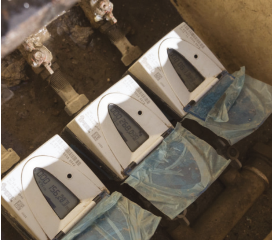
Figure 7. Example of an inspection pit in Gorino Ferrarese, Italy.
