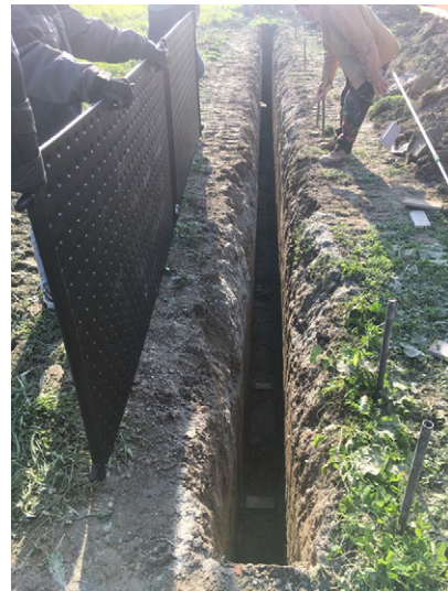
Figure 4. Flat-Panels and trench.
