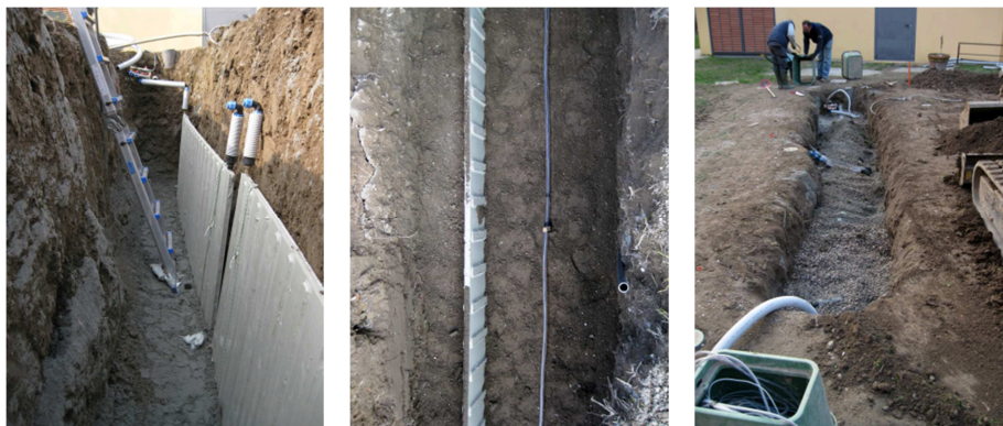
Fig. 2.5 The installation of Flat-Panels.
