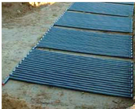
Fig. 1.6 New concepts of horizontal ground heat exchangers.
