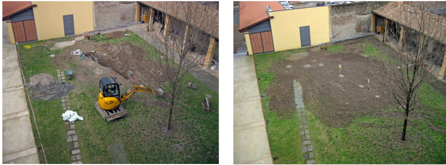
Fig. 2.6 The building after during installation and after.
