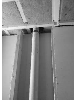
Figure 11 – Realization of waste water pipe inside a lightweight construction
