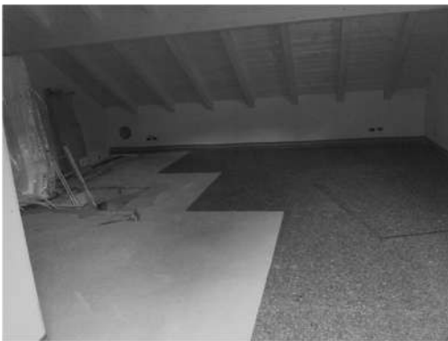
Figure 15 – second floating floor
