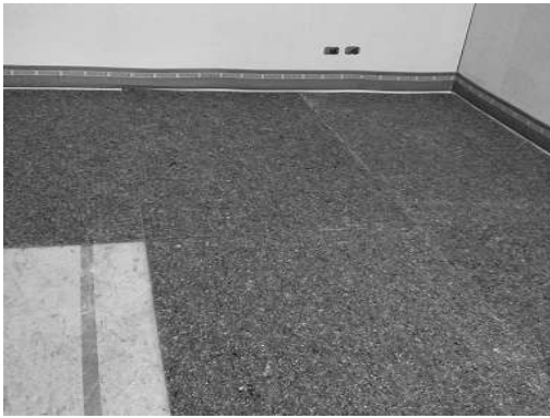
Figure 14 – first floating floor
