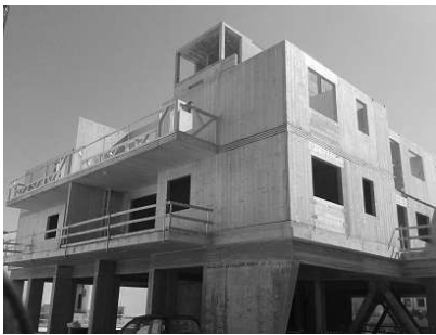
Figure 1 - multi-storey crosslam building
