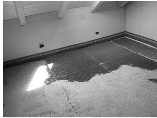
Figure 14 – first floating floor
