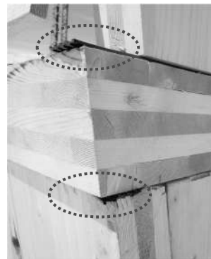
Figure 4 – wall-floor junction detail with elastomeric layer.
