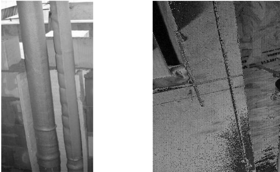
Figure 5 – Typical vibrant insulator for water pipes a) expanded PE, b) resilient ring
