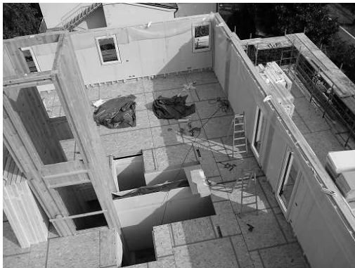
Figure 9 – multi-storey glulam with top boards building
