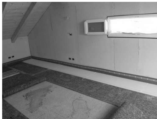
Figure 15 – second floating floor
