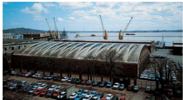
Figure 5: Seaport Deposit of Montevideo. Designed and built by Eladio Dieste in 1979 © Udelar Archives
