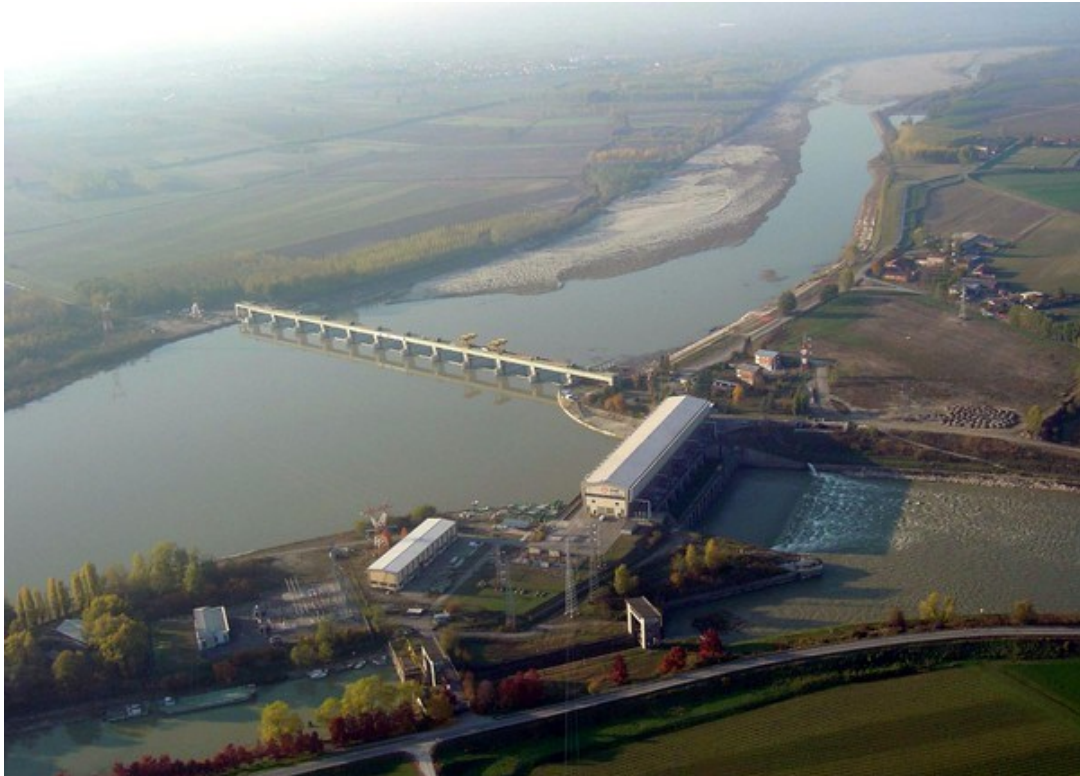
Figure 9. Aerial view of Isola Serafini run-of-river hydropower plant (flow upwards). The barrage diverts part of the flow to the power station on the right.
