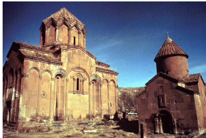
Figure 3.3. Southwest view from the Marmashen Monastery, 10 th -11 th Century ("Index of Armenian Art: Armenian Architecture, Marmashen," n.d.)
