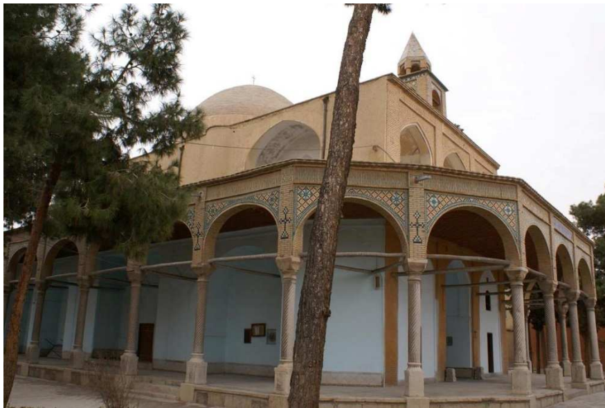
Figure 7.3. The church of Surb Astvatzatzin, the columns are decorated in the traditional Iranian style with bricks and polychrome tiles (The Armenians Community from Isfahan and South of Iran, 2014)
