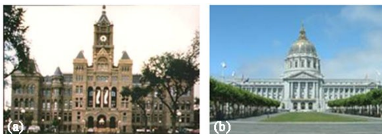
Fig. 4 (a) Salt Lake City & County Building (USA, 1894), (b) San Francisco City Hall (USA, 1912), (in Indirli, Martelli, 2009)
