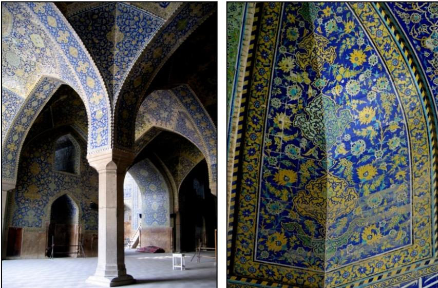
*Figure 1.2 Vast application of haft rang tilework at Masjid-i Jāme‘-i ‘Abbāsī of Isfahan (left) (photo: the author) and details of the polychrome tiles (right) (photo: courtesy of A.H. Karimy)*
