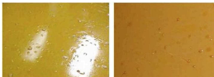
Figure 3.19: Photographs of defects on the linseed oil coating of a malfunctioning RPC.
