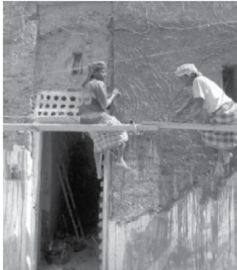
Figure 1 - Rehabilitation of mud tower houses
