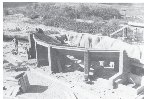
Fig. 16 - Original photo n.6, building of the concave shaped sliding surface (from GHETTI, 1962)
