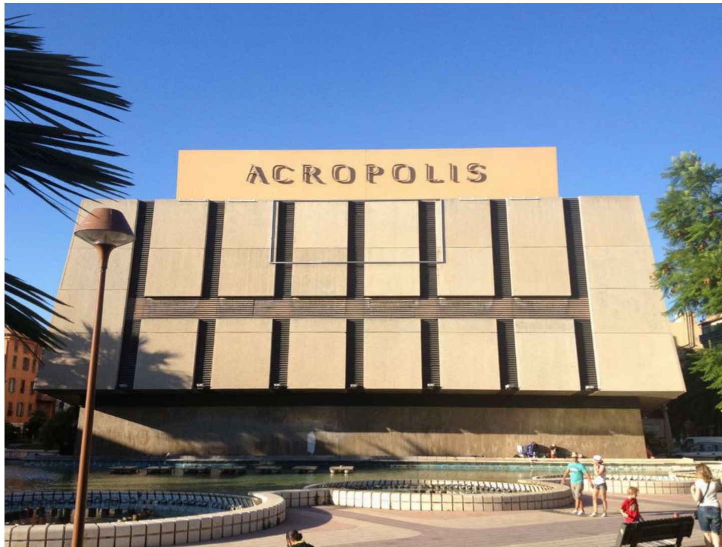
13. The southwest facade of the Multipurpose Center designed by G. Buzzi, P. Baptiste and P. Bernasconi (1981–1984) with consultancy on acoustic design by Prof. Eng. Lothar Cremer (formerly a consultant to Hans Scharoun for the Berlin Philharmonic) for the Auditorium. Photo credit: author, 2014
