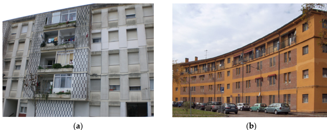
Figure 2. Typical post-war residential buildings in Italy. (a) Post-war building in Bologna made of prefab concrete panels, (b) building block in Ferrara built in the 1950s, made of a concrete structure and hollow brick blocks.
