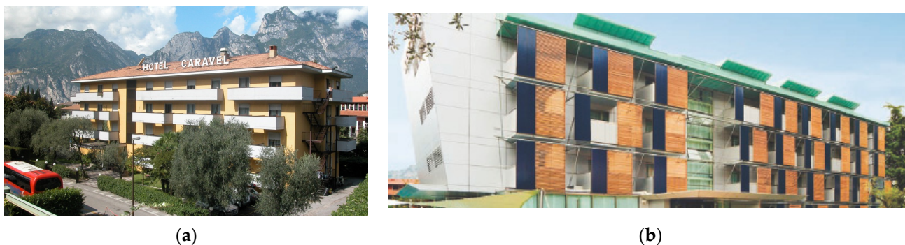
Figure 10. Refurbishment of a building block from the 1960s by adding solar shadings. (a) The building before the intervention. (b) The building after the intervention of adding wooden mobile solar shading on the south façade. This intervention contributed to a reduction in energy consumption for cooling of about 30%; moreover, the loggias can be used as additional living space.
