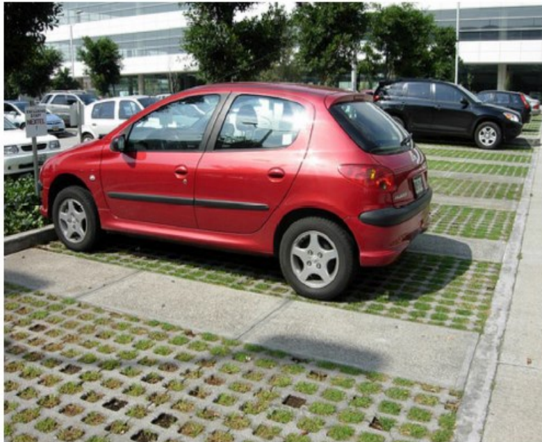
Figure 4. Porous surface in a car park.
