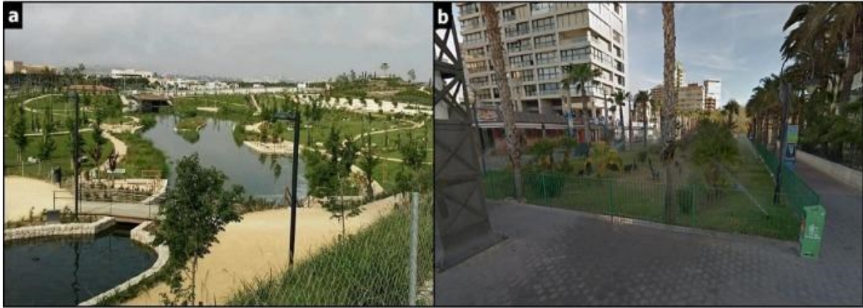
Figure 10. High-capacity rainwater collecting components incorporated into the urban setting, (a) Marjal Park in Alicante, (b) the final segment of Liriet Ravine in Benidorm.
