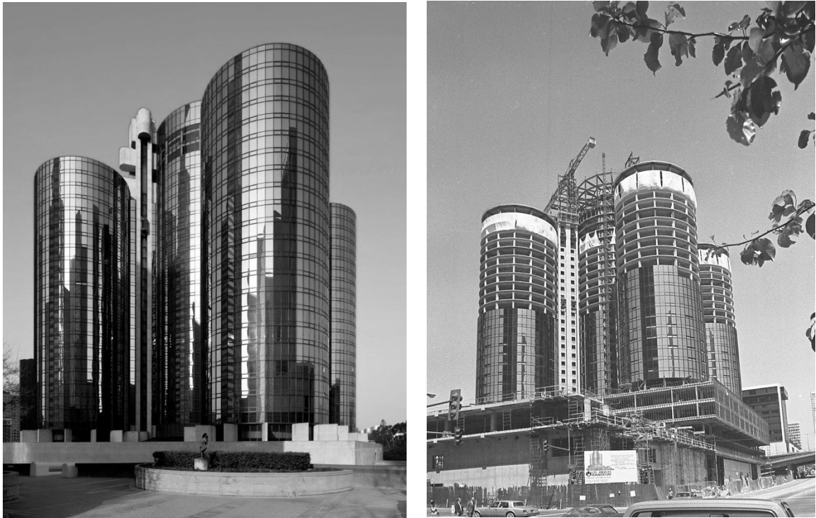
Fig. 3.26. John Portman, Westin Bonaventure Hotel , Los Angeles, California, 1974-1976 (source: https://www.skyscrapercenter.com/building/westin-bonaventure-hotel/4800 )
