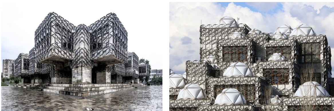
Fig. 6.14. Andrija Mutnjaković, The National and University Library of Kosovo, Facade , Prishtina, 1971-1982 (source: www.socialistmodernism.com ); Fig. 6.15. Andrija Mutnjaković, The National and University Library of Kosovo, Dome Structure , Prishtina, 1971-1982 (source: www.socialistmodernism.com )
