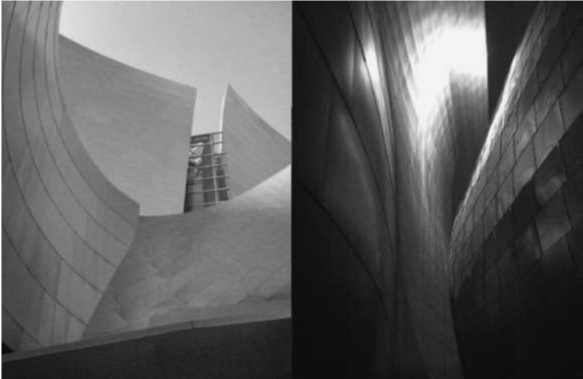
Figure 55 – Partial views of the Walt Disney Concert Hall in Los Angeles, designed by Frank Gehry (adapted from Llach, 2015, p.96)
