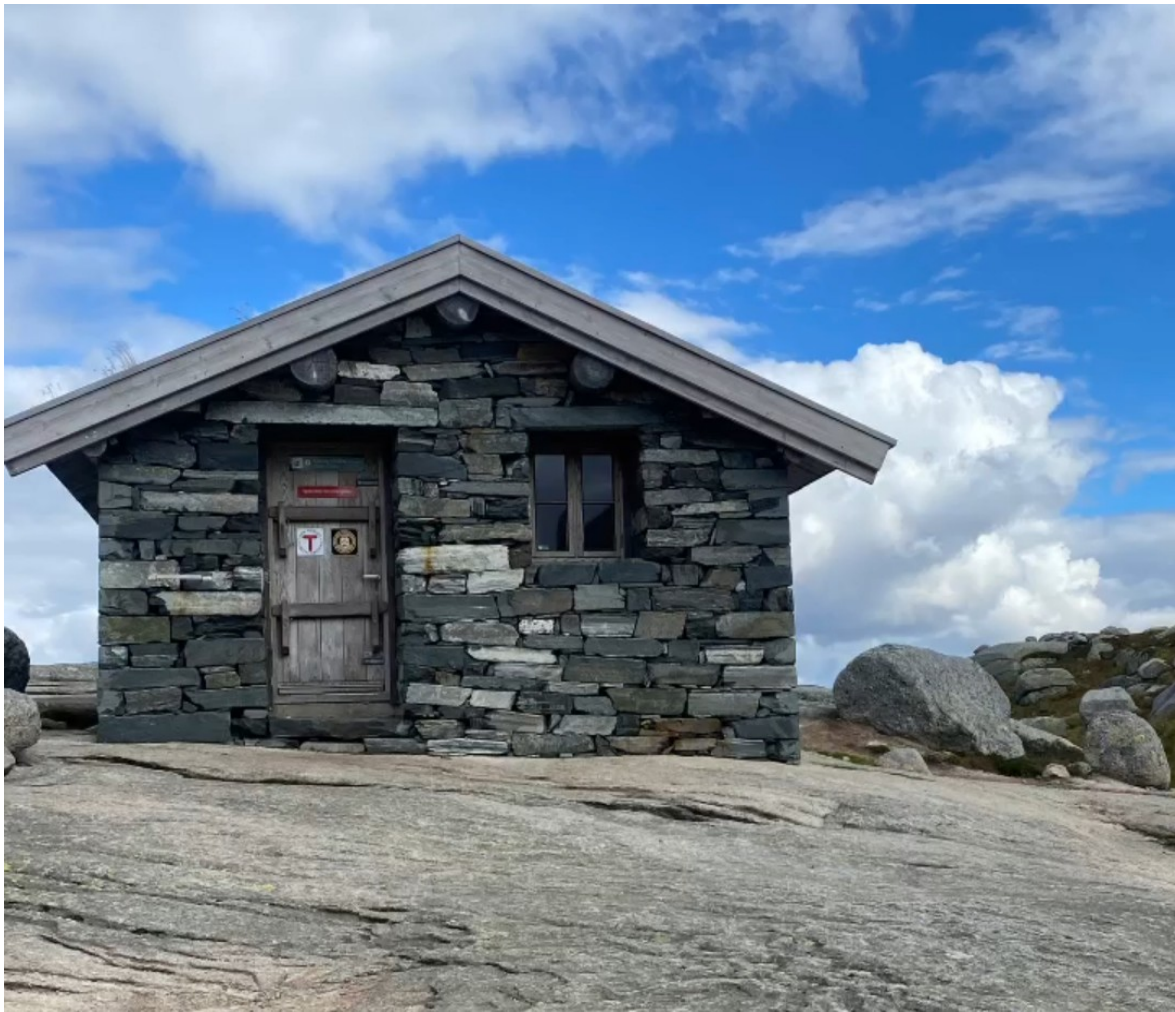
Figure 50 - Tectonic articulations, emergency cabin near Kjeragbolten, Norway (author, 2022)
