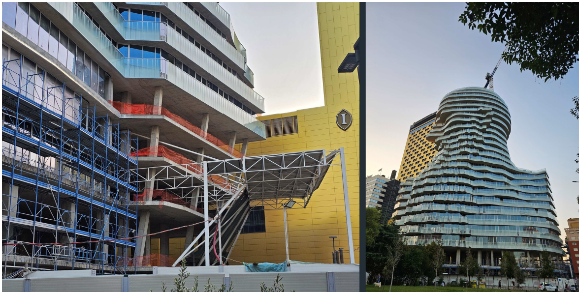
Figure 29 - Skanderbeg Head Building, spatial truss for “Skanderbeg’s shoulder”
