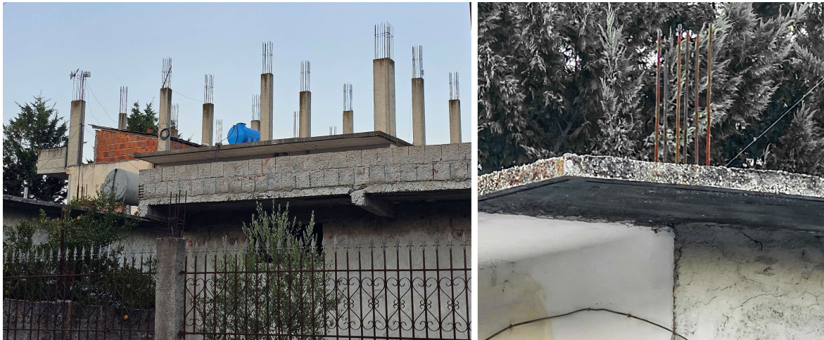
Figure 30 - Bars and unfinished structures over terraces (author, 2025)
