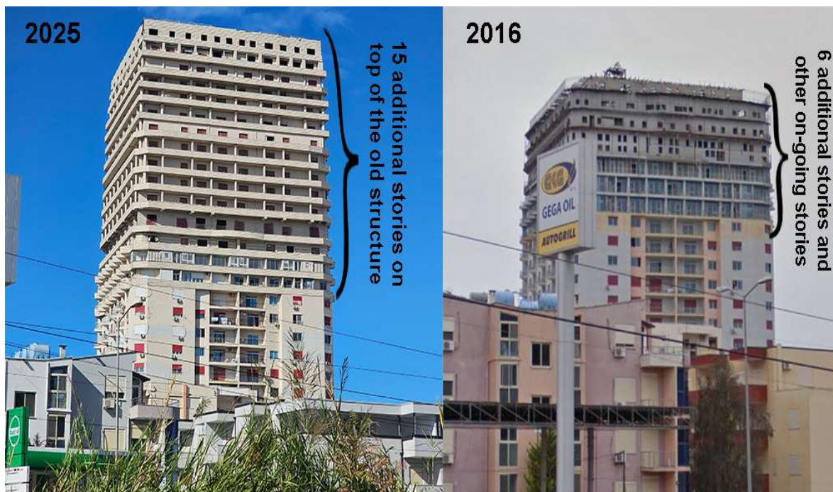
Figure 48 - A building in Durrës with 15 additional stories above the old structure (author, 2016&2025)
