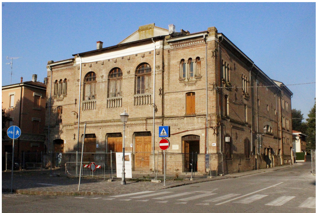
Fig. 2. View of the main façade of the Theatre of Novi along Via dei Martiri della Libertà. Photographic survey, July 2020. Photo by M. Suppa.
