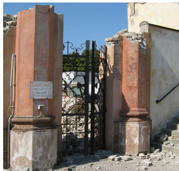
Fig. 6-7. Details of the entrance overturning. Ph Arch. Pedrini.
