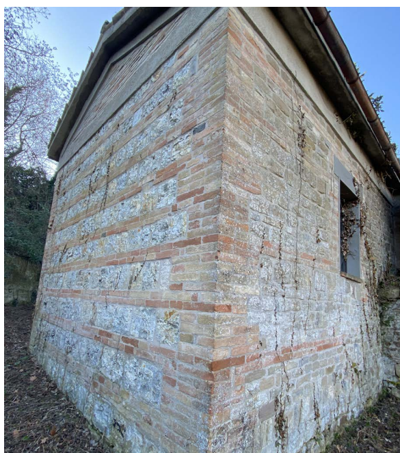
Fig.21. Cemetery of Pallino (PU). Masonry in brick and stone. Ph Archaeologist Siegfried Vona
