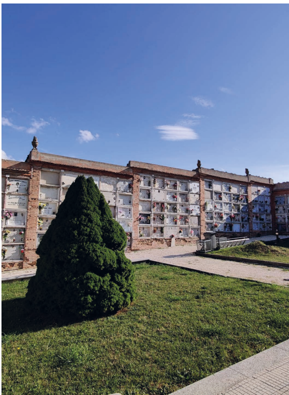
Fig.2. Cemetery of Poggio Cupro (AN). Columbaria without porch built on sloping ground. Ph Arch. Marta Zannotti
