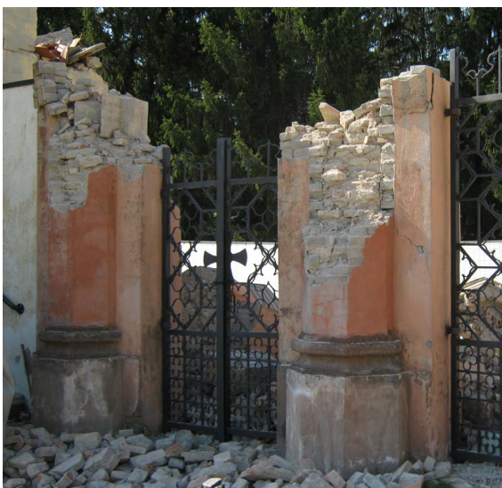
Fig. 6-7. Details of the entrance overturning. Ph Arch. Pedrini.
