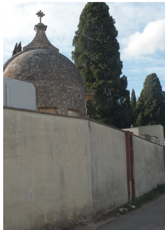
Fig.3. Cemetery of Grottaglie (TA). Family tomb with non-trusting roof but high projecting elements. Ph Riccardo Annicchiarico
