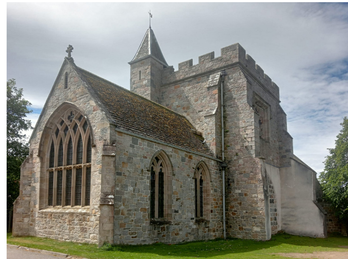
Fig. 8.38. Picture of St Margaret's Church in Braemar, showing exterior surfaces in granite masonry.
