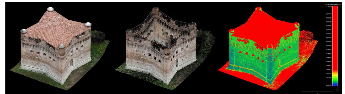
Fig. 6.03. RGB data of laser scanner point cloud obtained through reprojection from photogrammetric point cloud in Rocca Possente in Stellata dataset. Original photogrammetric point cloud (right), colorized laser scanner point cloud (middle) and cloud-to-cloud distances (left). Red areas show distances bigger than 2cm, note that shadow cones in façades and the roof, not acquired thorough terrestrial laser scanning, and noise surfaces, such as grass.
