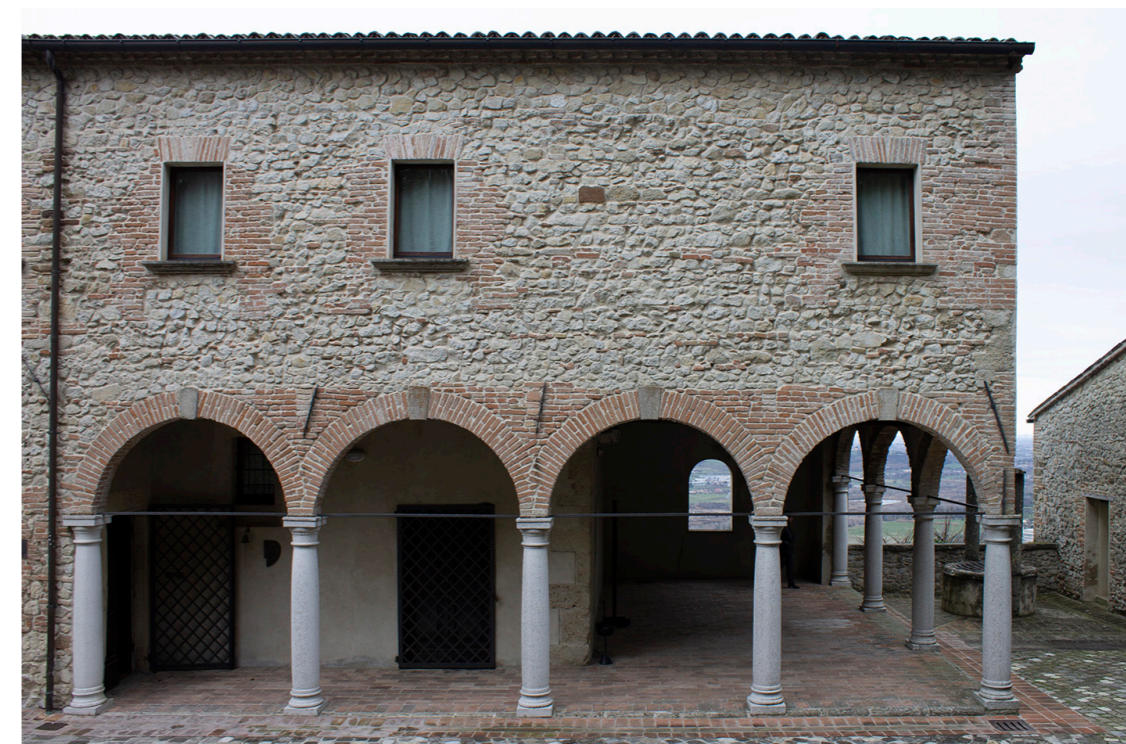
Fig. 6.08. Detail of the materials of the external surfaces of the Former Monastery of St. Agostino in Verucchio.
