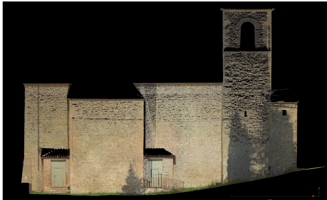
Fig. 6.02. RGB data of laser scanner point cloud obtained through onboard camera in BLK360 in Former Monastery of St. Agostino Verucchio dataset. Colour difference between light and shadow areas are observed.
