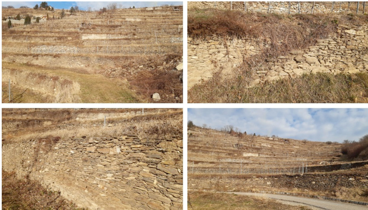
Figure 5. Details of the dry stone wall terraced area CH2 (credits to Rainer Vogler).
