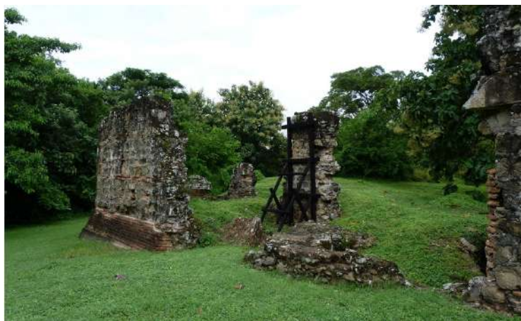
Figure 2. Walls of the Casas Reales Complex. The bottom part still shows the erosion due to the tides “carving” effect.
