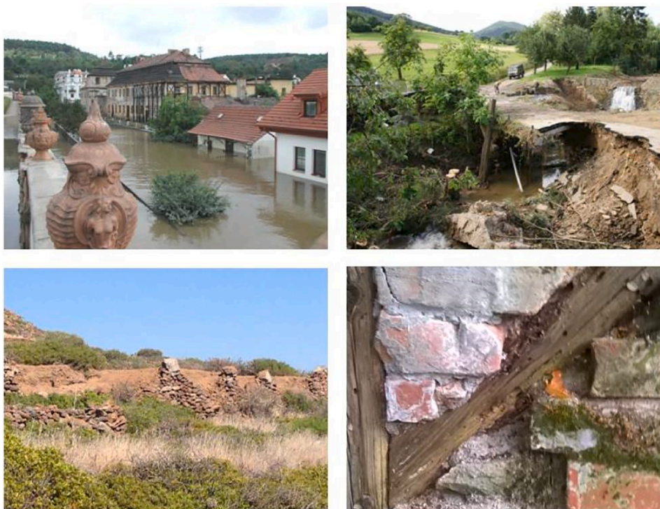
Fig.2. Examples of damages: top left, flooding in historic centre (photo: Drdácý); top right, heavy rain damage in Klingfurth (photo: Austrian Armed Forces, 2009); bottom left, erosion and partial collapse of dry stone walls in the Island of Filicudi, Aeolian Archipelago (photo: Sardella); bottom right, water damage to half-timbered wall (photo: Cacciotti, 2015).
