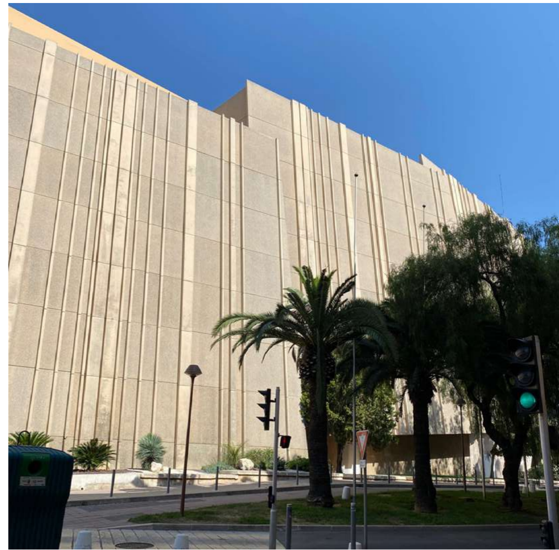
16. Detail of the exterior facades of the Auditorium. The precast reinforced concrete facades with irregular vertical reliefs were found to be articulately sloping inward toward the building, creating a sharp discontinuity from the surroundings. Photo credit: author, 2017
