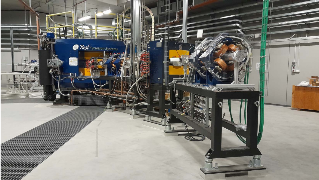
Figure 3: Picture of the cyclotron in its room at the SPES building.
