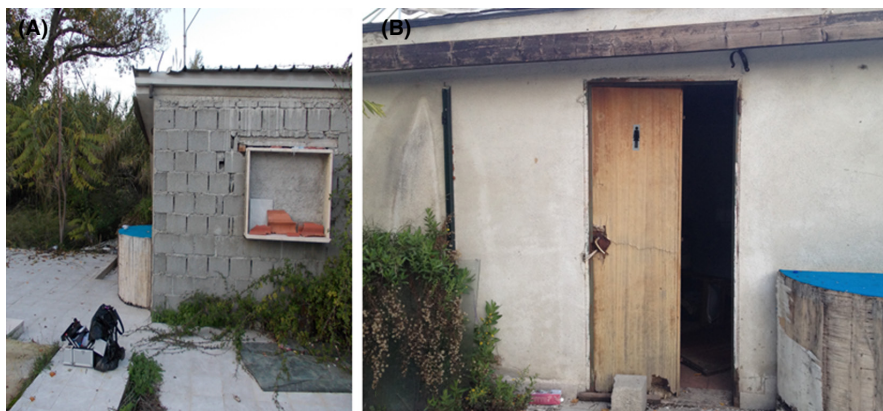
FIGURE 1 Abandoned sport facility in a suburban area near Cosenza (Calabria, Southern Italy) where the body of a 50-year-old man was found. (A) External view. (B) Open door for access to the building [Color figure can be viewed at wileyonlinelibrary.com ]
